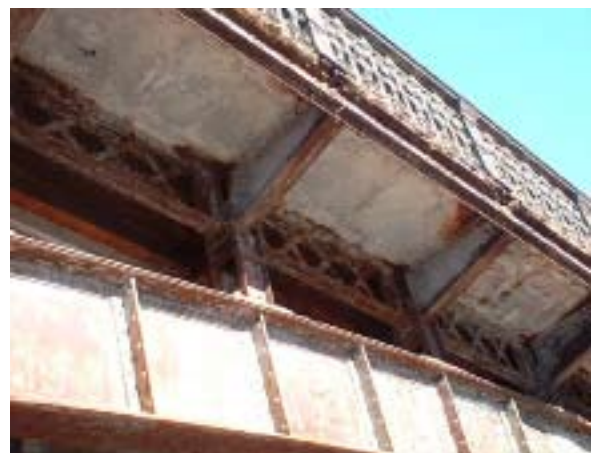
Figure 4: Beams (perpendicular to bridge) and Stringers (sections with “x” bracing) (Source: DCR 2006 Inspection Report)
