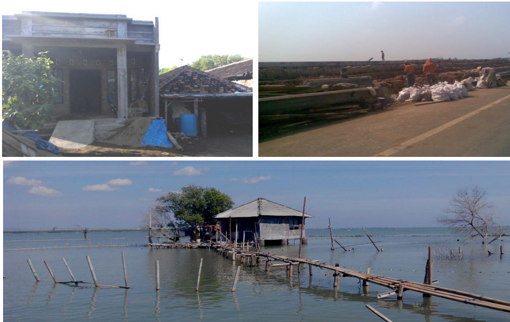
Fig. 8. Adaptation have been created against the slow disaster of sea inundation from climate change impact and others influence factors by increased the houses, elevated the road, and survived the house like “a private place” at the sea.
