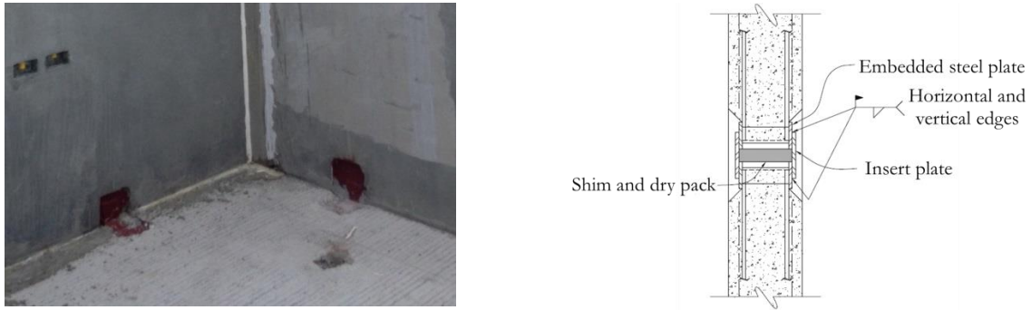
Fig. 6. Connection detail of Welding of steel plate embedded in precast concrete wall and insert plate.
