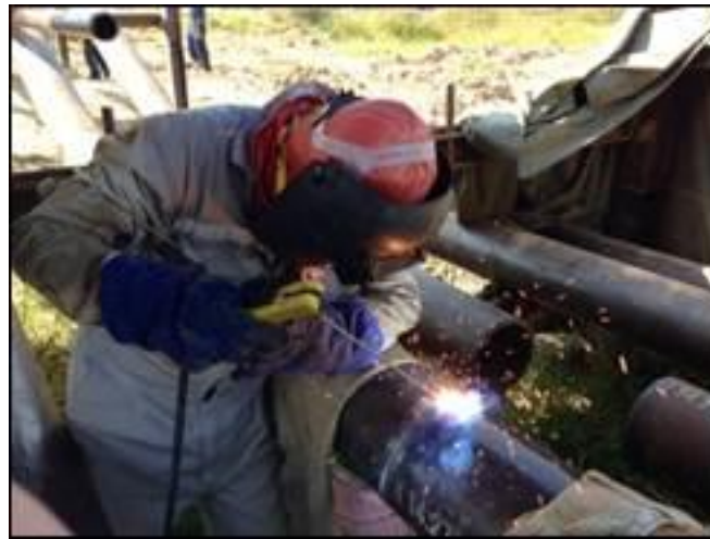
Fig. 1. Pipeline maintenance at an onshore crude oil transportation pipeline site.
