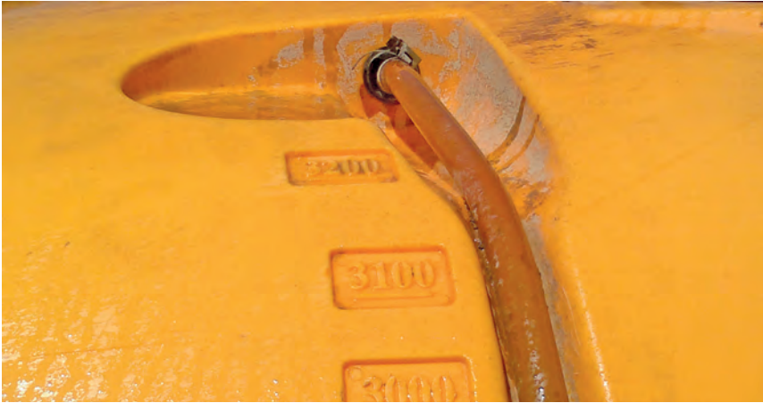
Fig. 3. Useless tank level indicator.
