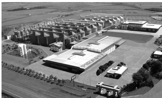
Figure 1 Receiving, drying, storing and processing rice facility in São Borja, State of Rio Grande do Sul, Brazil, where the Rice Quality Program is being applied, since April 2008.
