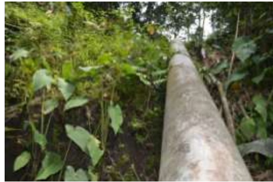
Gambar 6. Pipa Pesat (Penstock)
