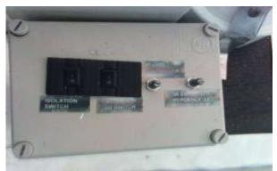
Fig.21. Solar circuit and emergency alarm circuit box
