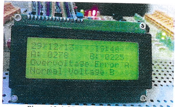
Figure 12: LCD Display at RTU Board
