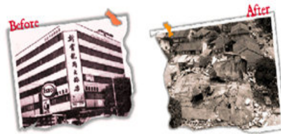
Fig. 3: Before and after the building collapsed.
