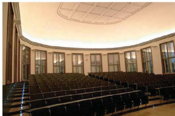
Fig.1. The implementation of MPP as a sound absorber in front of the window at University Freiburg lecture hall [6]
