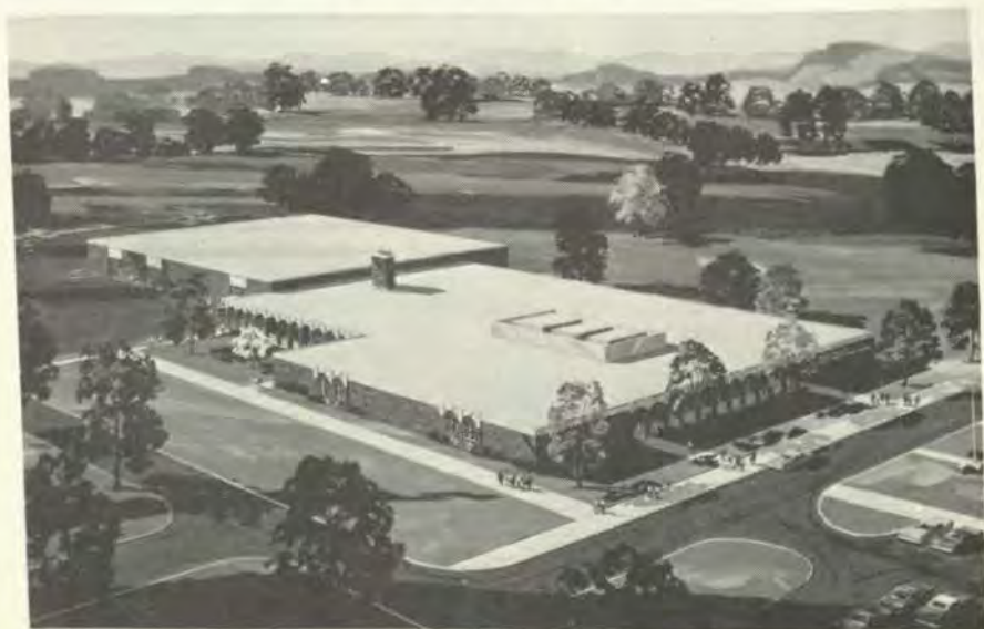
KNOX COUNTY JOINT VOCATIONAL SCHOOL
