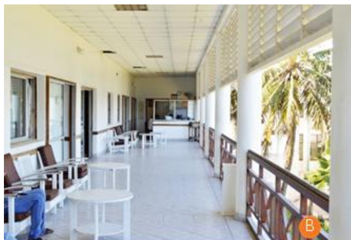
Figure 5. Reviewing sustainable site planning with natural ventilation.
