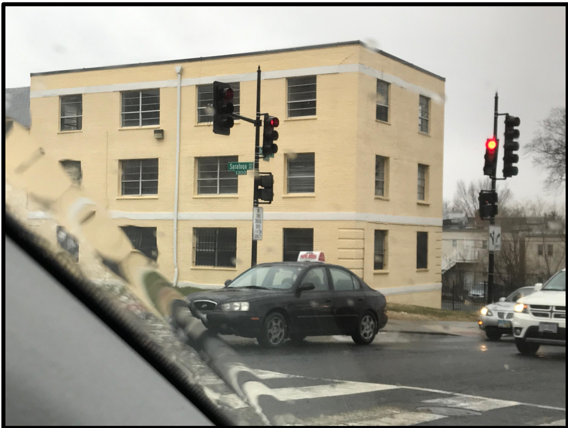
Figure 4. Brookland Manor Apartments. Empty, residents evicted. Photo taken by author, 2017.
