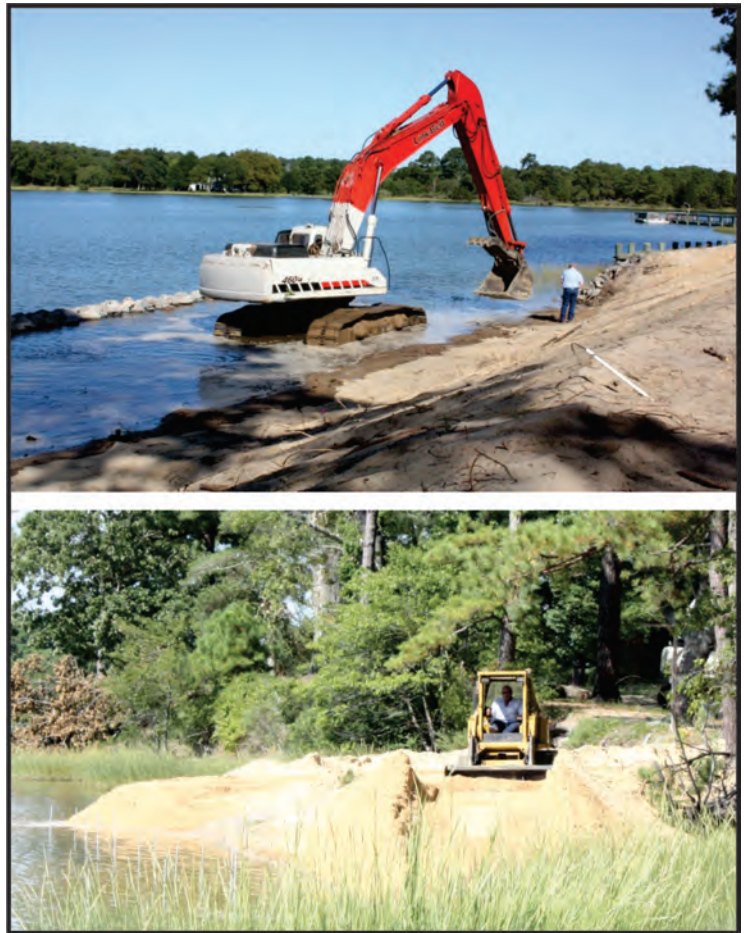
Figure 5-5. Construction of the shore structures at Occohannock on the Bay.
