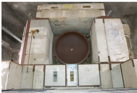
Figure 19: The NuMI Beam Hadron Absorber. The top Figure shows a schematic of the hadron absorber. The left bottom picture shows concrete block shielding around the downstream end of the decay pipe before the installation of the hadron absorber. The bottom right photograph shows the completed hadron absorber with the back wall of concrete blocks, and the steel roof blocks.
