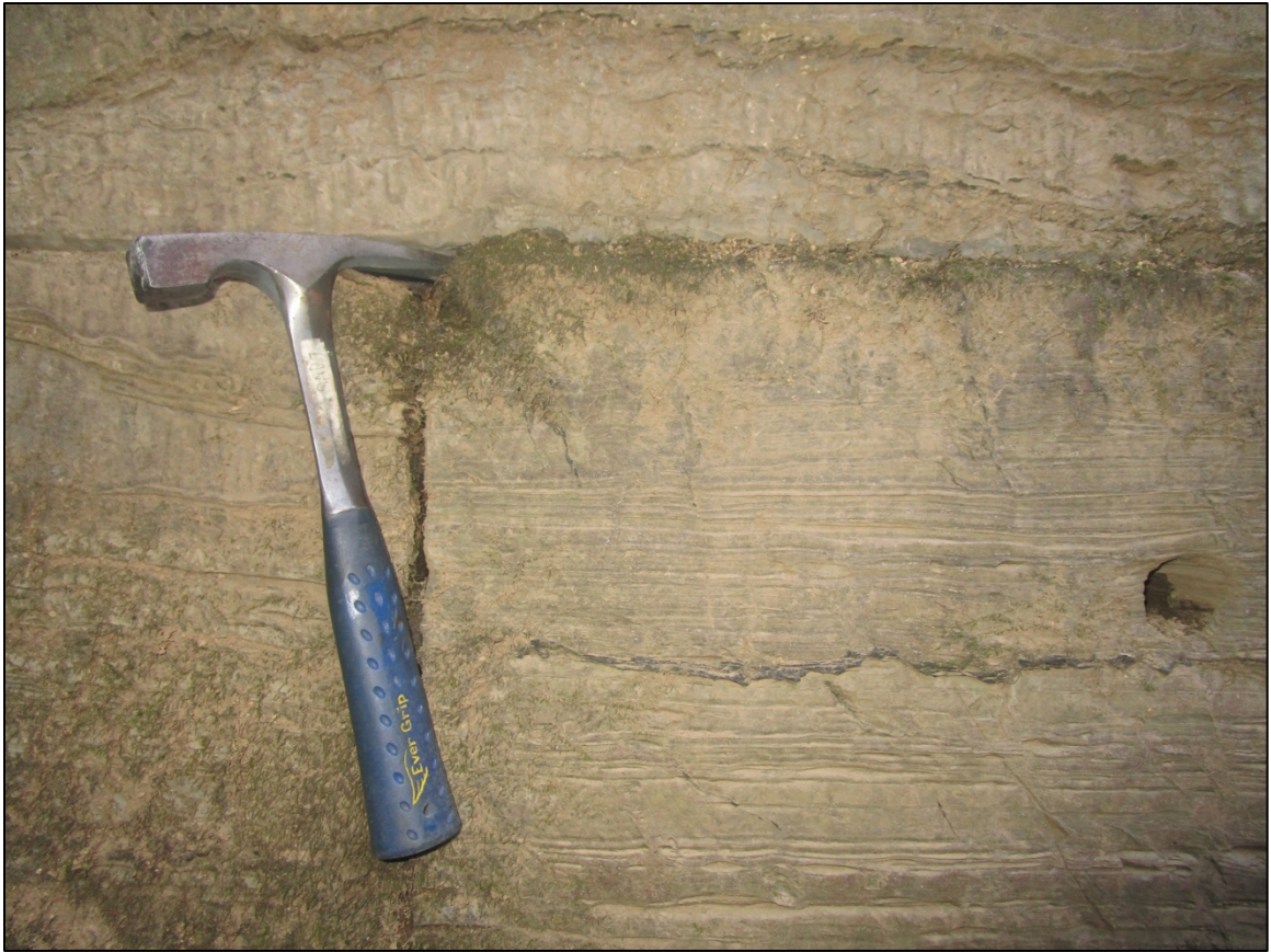
Figure 45. Cambrian-Ordovician limestone from the rock facing over the western portal of the BRT.
