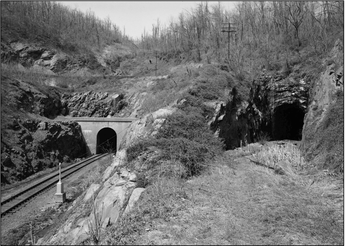
Figure 4. Eastern portals of the new and old Blue Ridge Tunnels, respectively. Photograph from 1968. Image from the Library of Congress archives: https://www.loc.gov/item/va0254/ .
