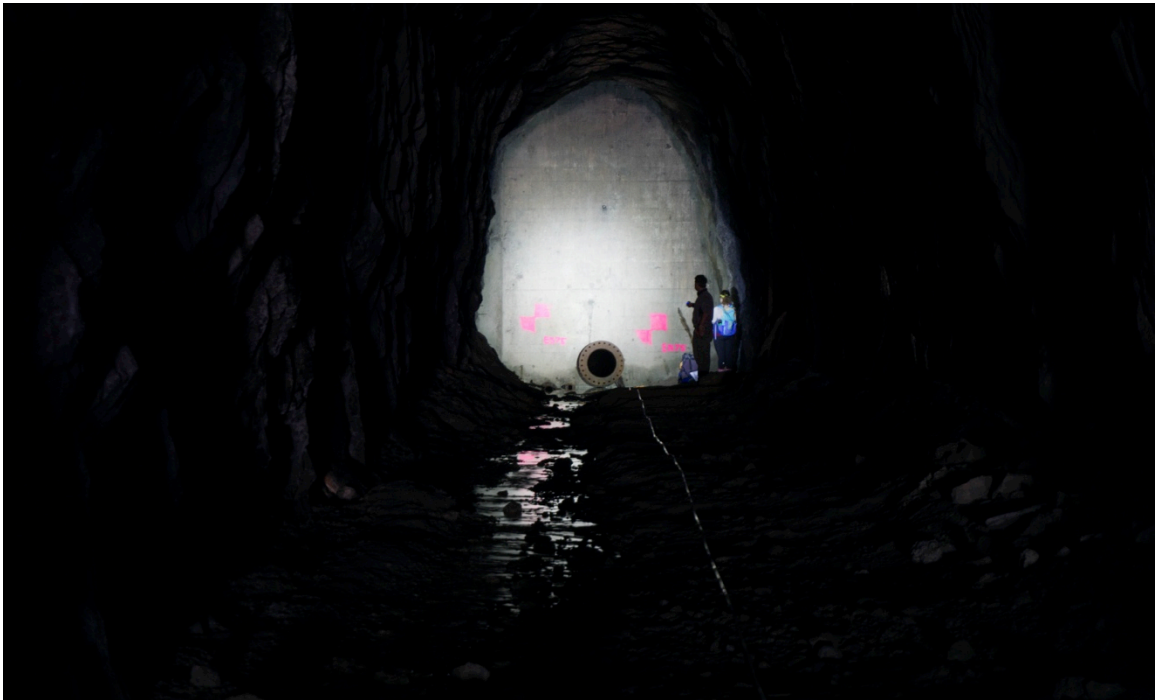
Figure 16. View from the eastern portal of the Blue Ridge Tunnel looking towards the concrete bulkhead 750 feet (230 m) inside the entrance. Note the water on the tunnel floor and the tube that provides the only access to the middle of the tunnel.
