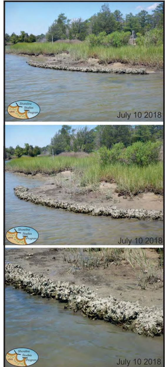
Figure 4-27. Site 6 oyster bag sill two years after installation. The sill has provided shore protection and created habitat. A great many oysters are growing on the bags. In addition, sediment has come in behind the sill, the marsh is no longer scaped, and marsh grass runners are extending toward the sill.
