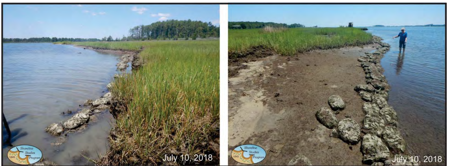
Figure 5-10. The 3-bag sill tended to remain intact when placed close to the eroding marsh scarp (left). However, when the bags are placed at low water farther from the shore because of the gentle slope of the intertidal area, they tended to roll.
