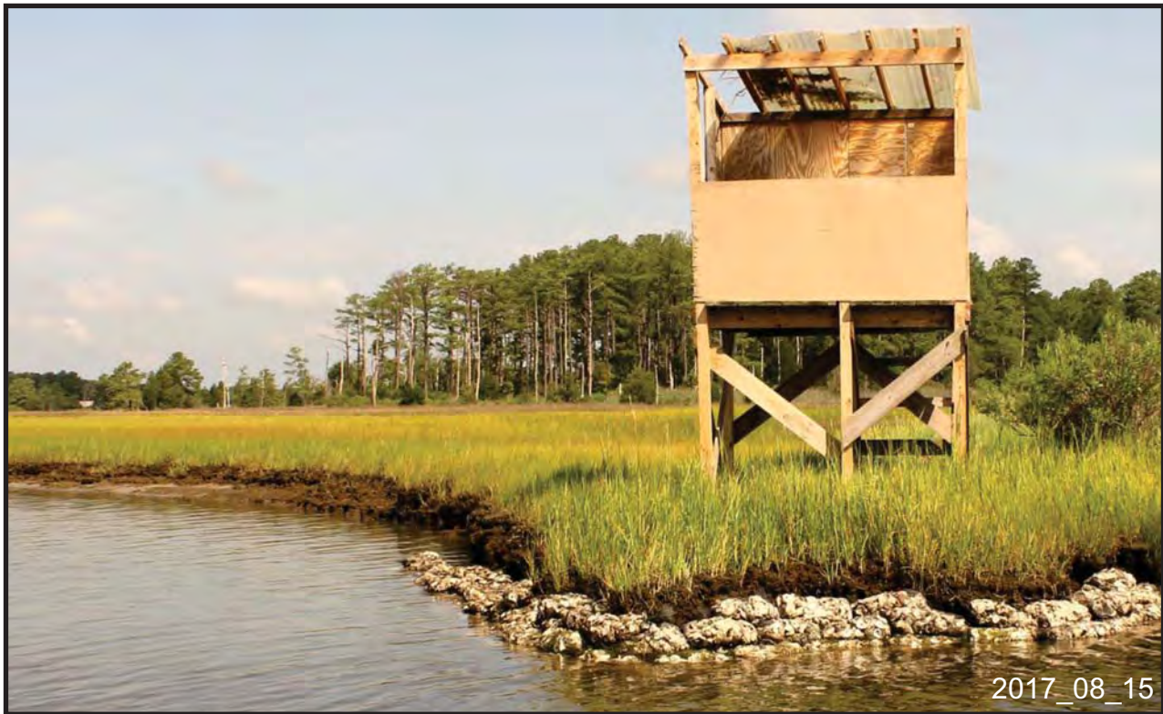
Sill 3 wraps around the point and comes in close to the marsh scarp to provide the maximum amount of protection to the shoreline. Photo credit Linda Tjossem.
