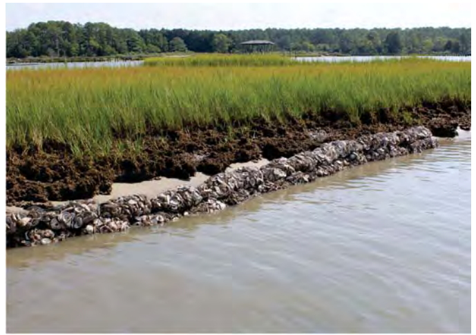
The finished sill along one section of shoreline and eroding marsh. Photo credit Linda Tjossem.
