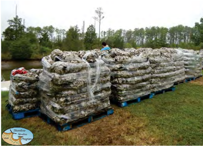
The 2,000 oyster bags were brought to a staging site by truck on pallets.
