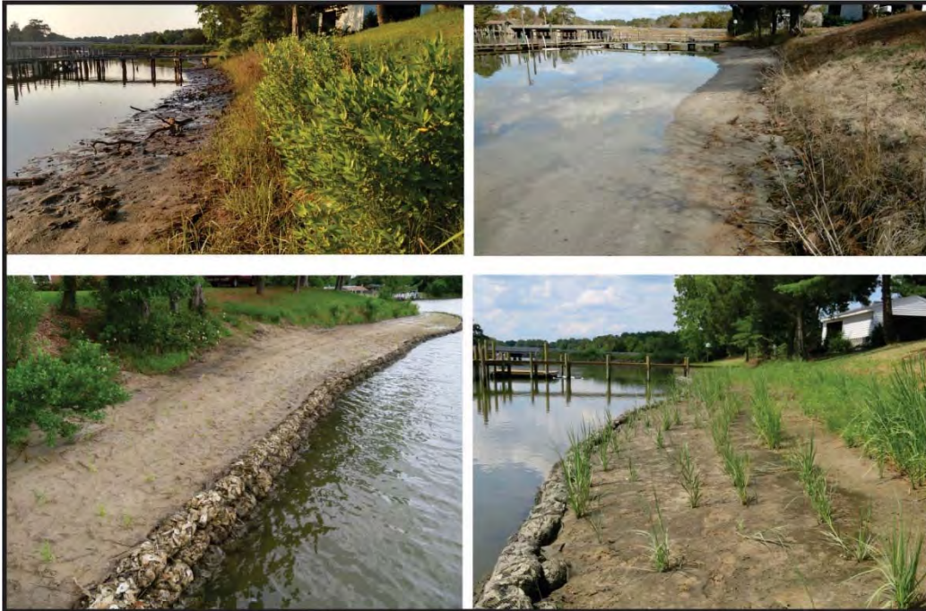
Figure 4-17. Site 4, Top left: Shoreline prior to the project on 26 May 2016; Top right: May 2017 prior to the bags being placed; Bottom left: after bags were placed in May 2017; and lower right: after the grass was planted in July 2017. Photo credit: Walter Priest.
