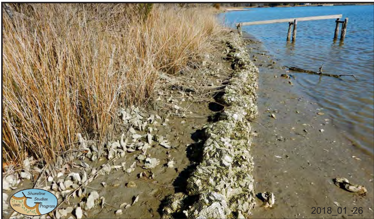
Sill 2. Some fine-grained sediment has been deposited behind the sill structure.
