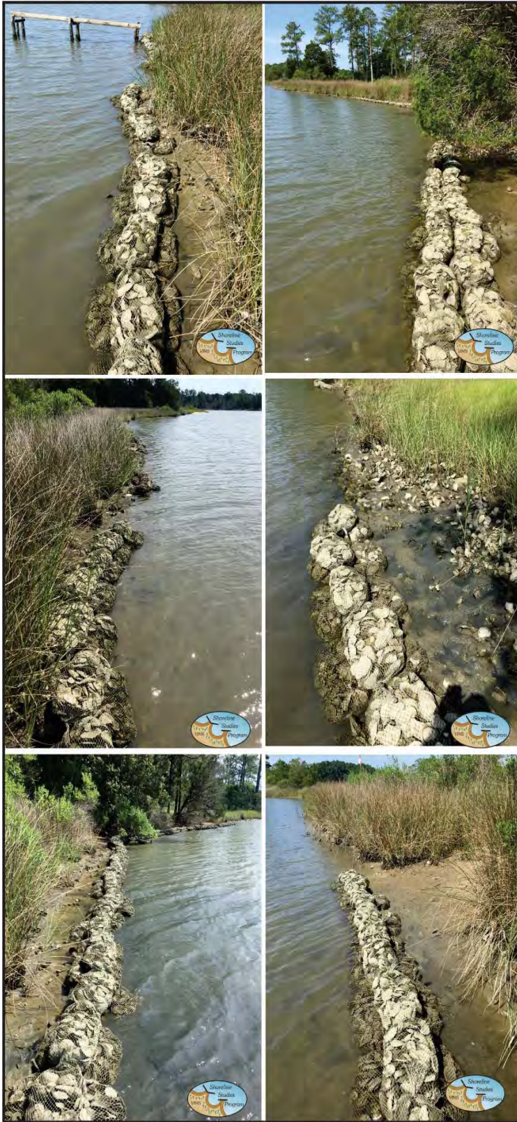
Figure 5-4. Heritage Park three months after construction (June 29, 2017).
