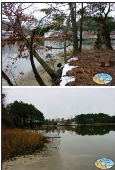
Figure 4-3. Site 1 before project installation. The marsh is eroding and an upland bank is exposed and eroding. Photo credit: VMRC permit application uploaded 28 Oct 2010.
