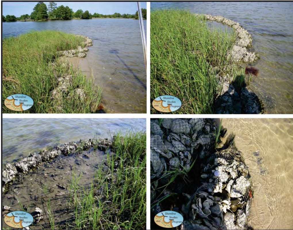
Figure 4-14. Oyster bag sill at Site 3, St. Johns Point on 10 May 2017 approximately 3 years after placement.
