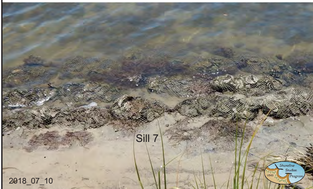
Sill 7 also had bags that rolled toward the marsh. Next to the headland, where the sill is closer to the marsh, sediment has been deposited landward of the bags.
