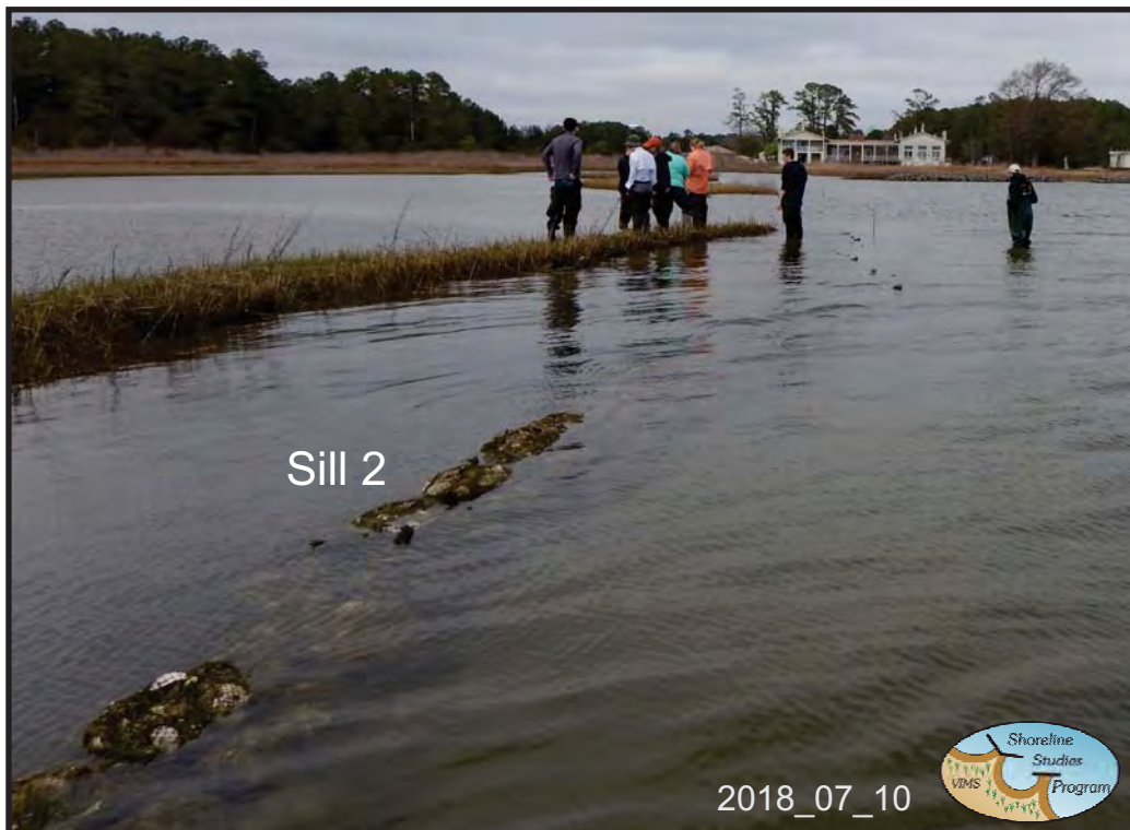
Sills 1 and 2 are 6 bag sills on the east-facing shoreline that fronts narrow, low marsh barriers that are covered at high water.
