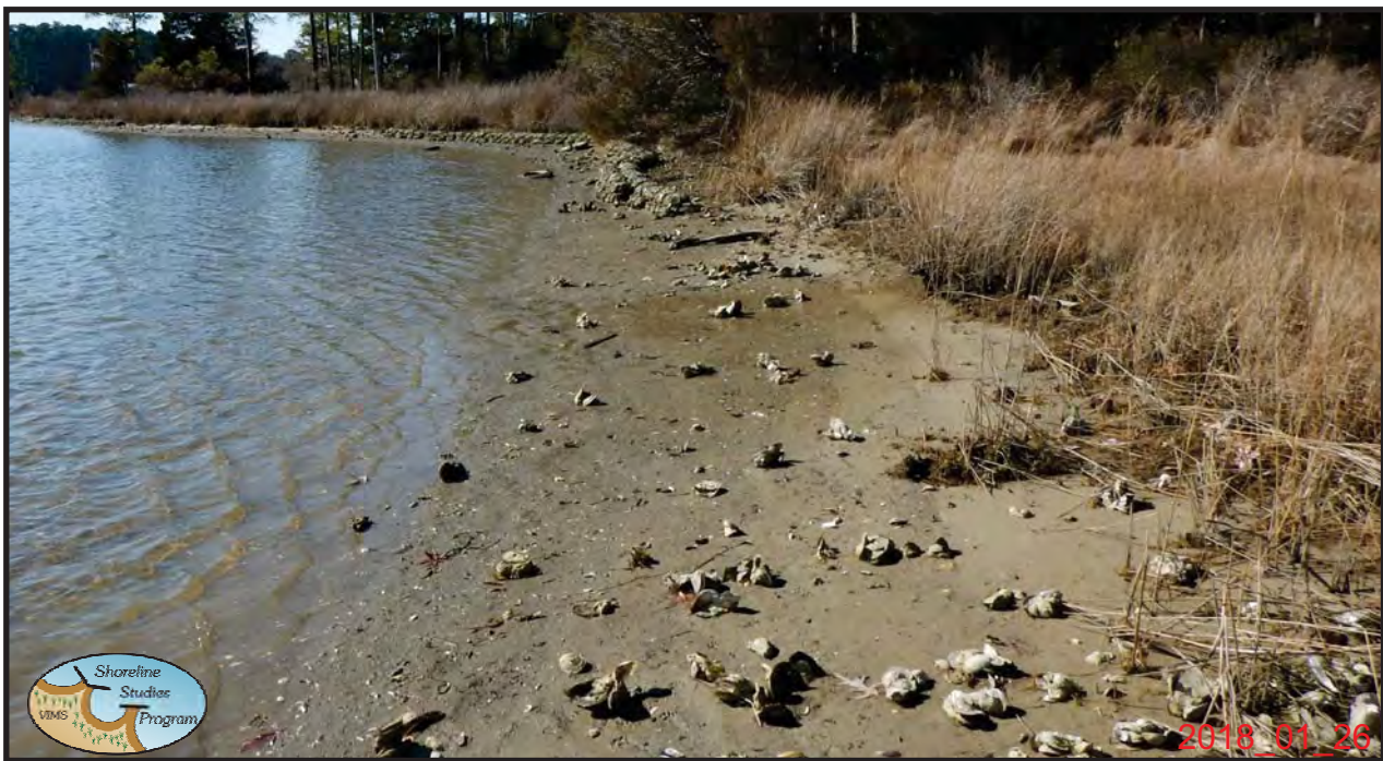
The shoreline between Sill 2 and 3 in the marsh looking toward Sill 3.
