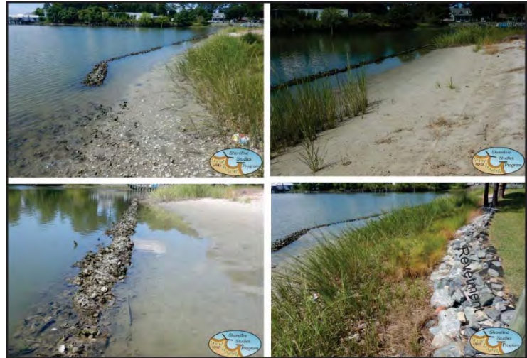
Figure 4-6. Present condition of Site 1 oyster bag sill (6 September 2018).
