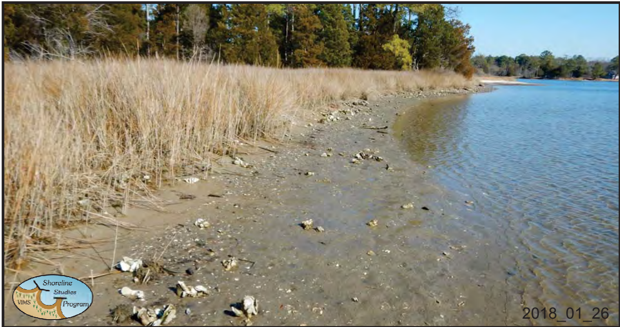
Looking north from the Sill 1 at Heritage Park.
