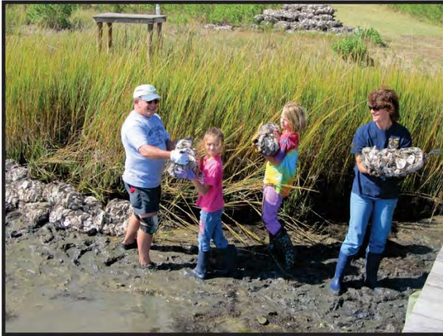
Figure 4-11. Placement of bags along the shoreline. Photo credit: Walter Priest, 14 Oct 2012
