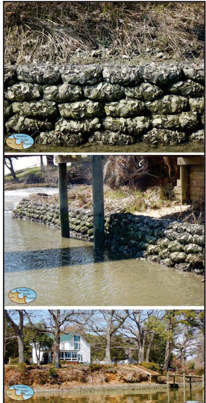
Figure 4-24. Site 5 on March 28, 2018. After nearly two years, the bags are still intact and have stayed as placed. Marsh has filled in behind the structure. Oysters have been recruited along the sill.
