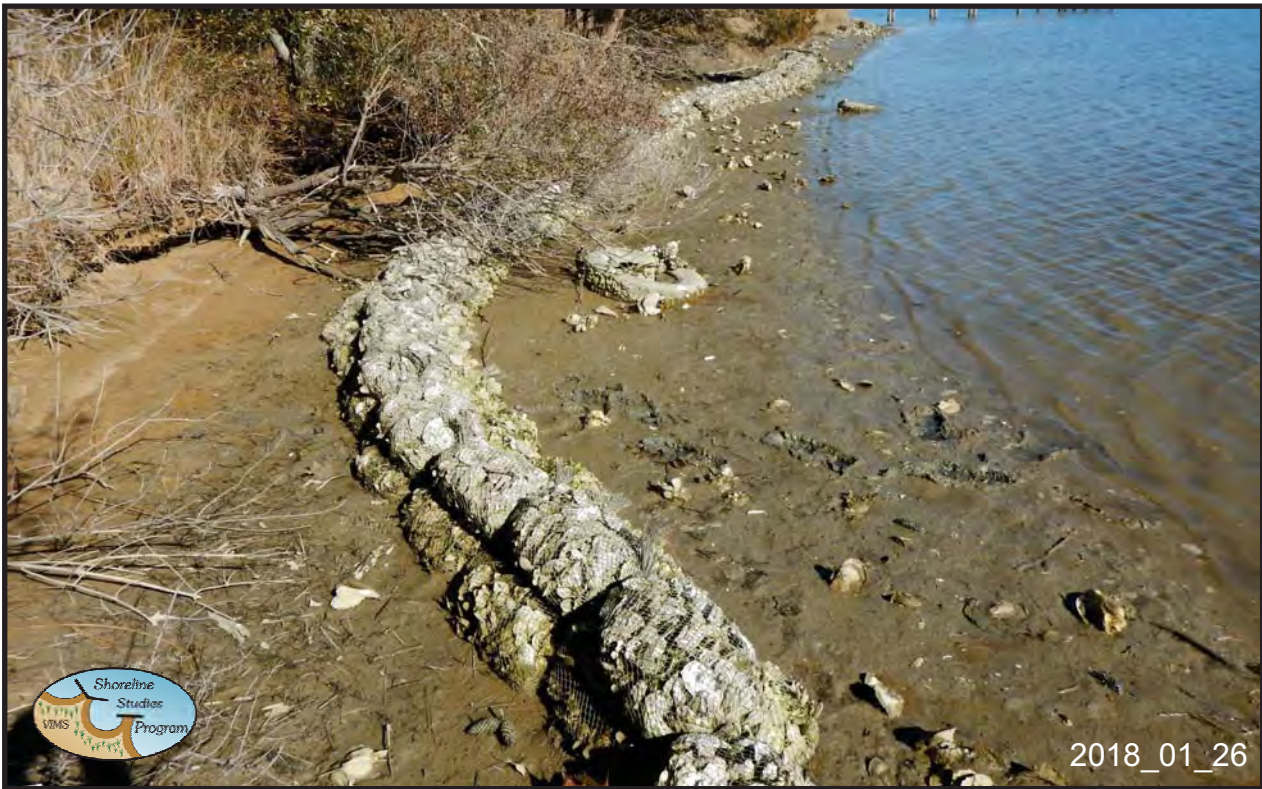
The southern end of Sill 3 flares out to follow low water.
