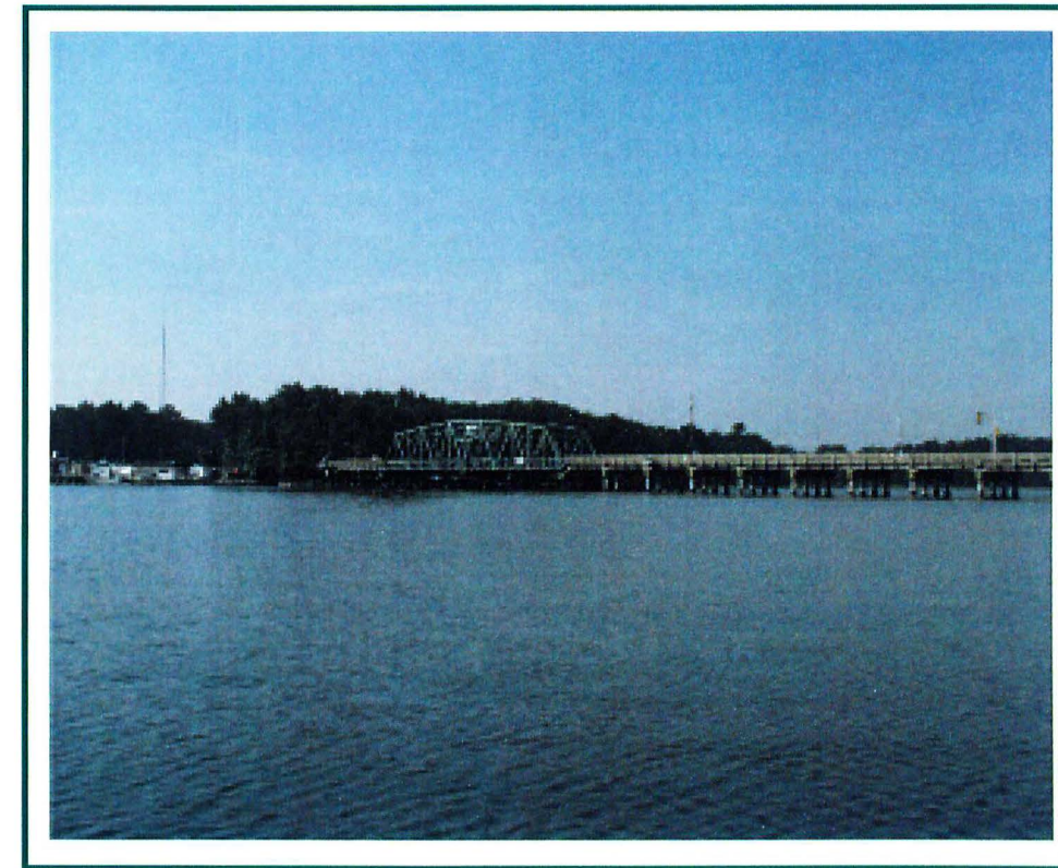
Bridge over Milford Haven to Gywnn Island
