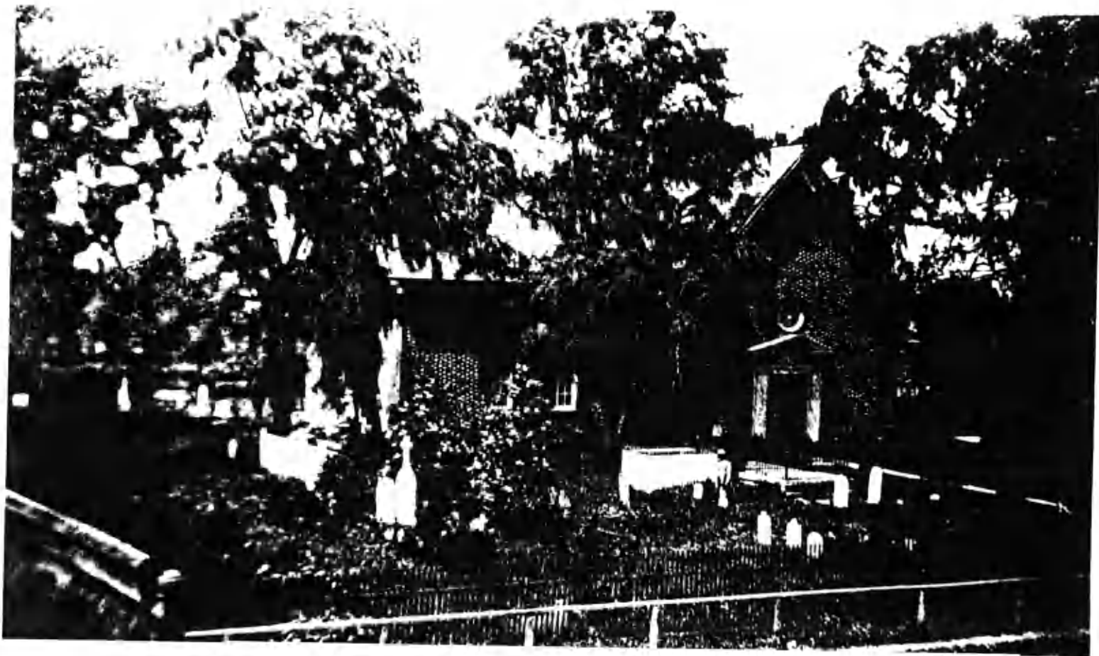
Plate 5b Portion of the west wall soon after 1892 and before 1901. Also, the iron fence on the south has been put up (1892).
