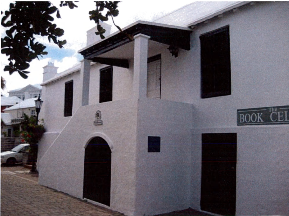
Figure 5 Photograph of the Tucker House Exterior.
