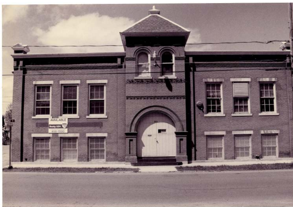
Figure 14. Now vacant plant of the Glens Falls Paper Box Company at 230 Maple Street.
