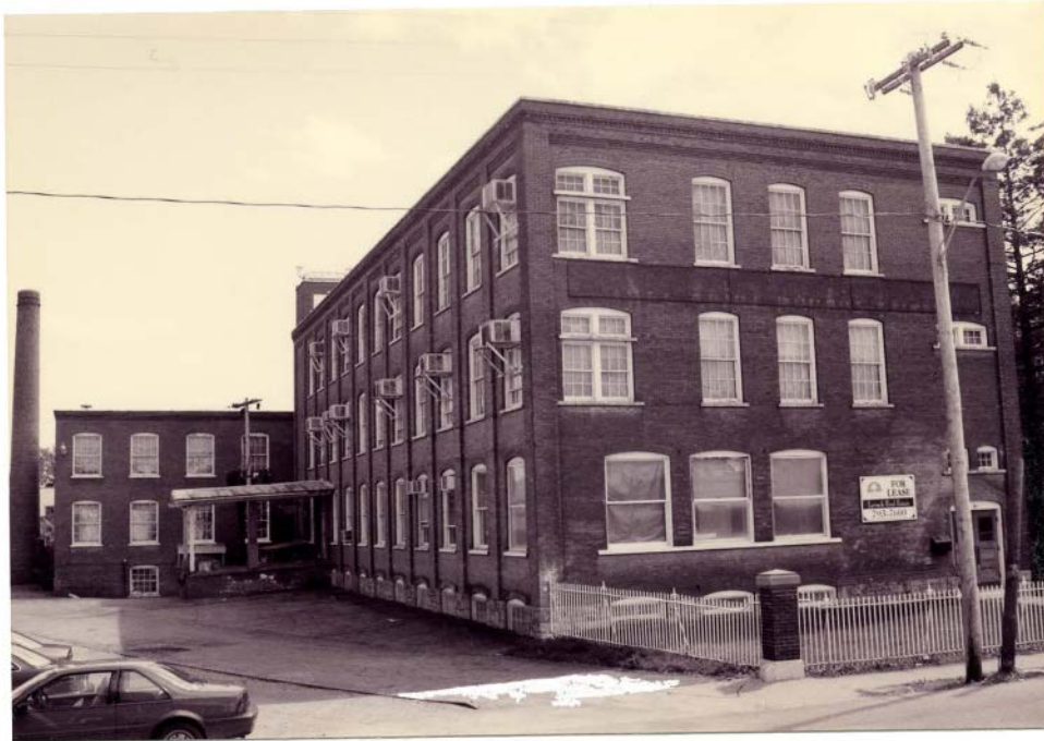
Figure 7. The now vacant mill of the Troy Shirt Makers Guild, Inc., and the former McMullen-Leavens Company at 71 Lawrence Street.
