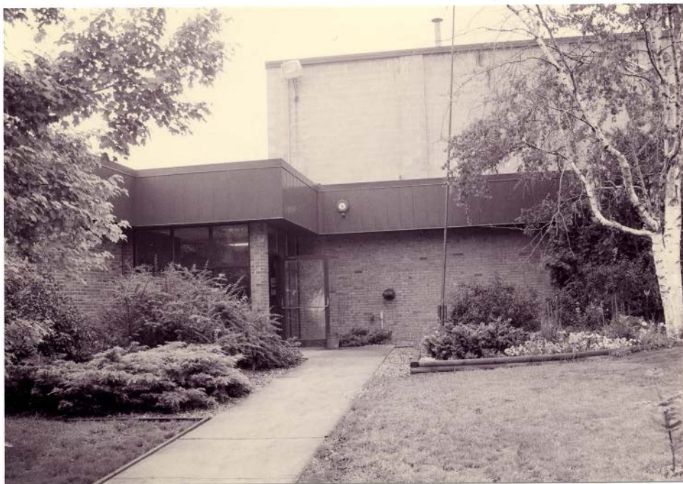
Figure 12. Ames Goldsmith Corp. building at 21 Rogers Street rebuilt in 1968.
