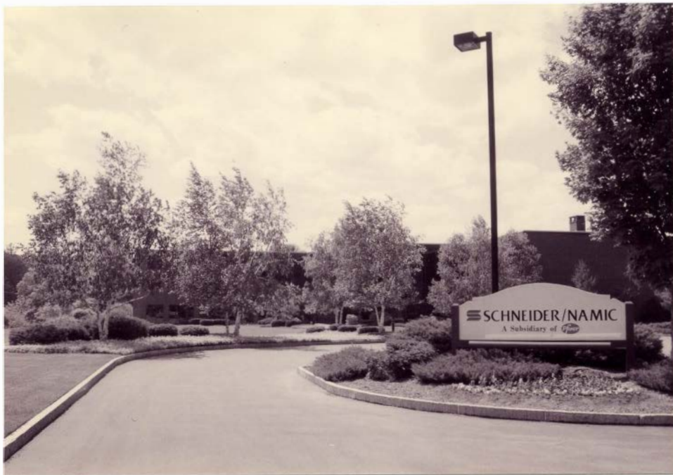
Figure 4. SCHNEIDER/NAMIC headquarters building located in Pruyn Island Industrial Park.
