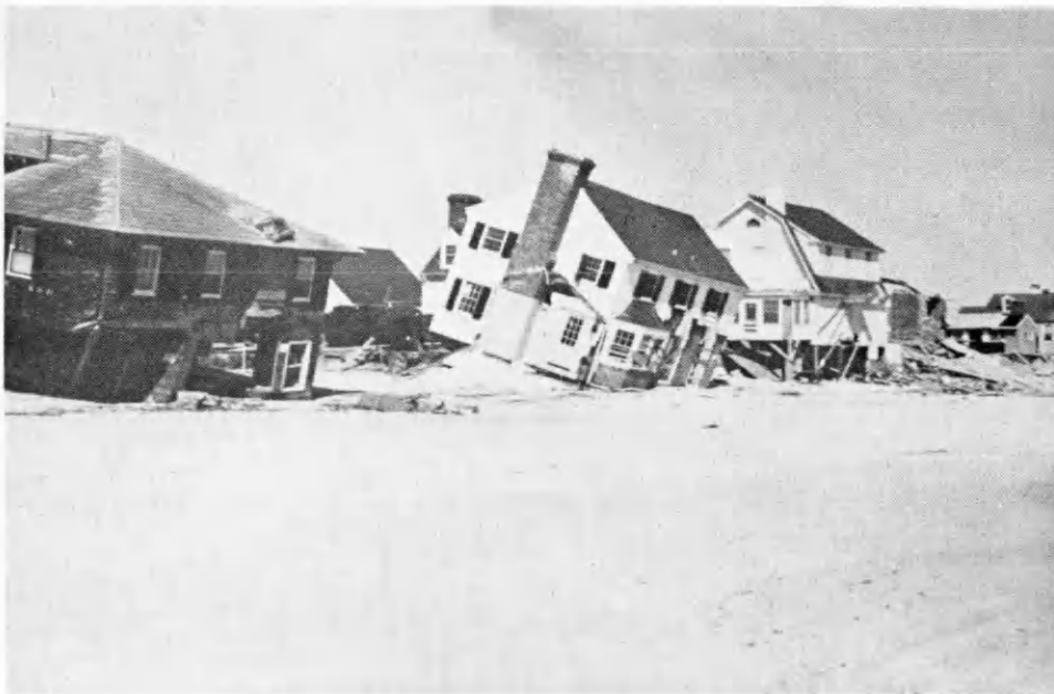
Figure 7. Photograph of property damage at Virginia Beach, Va. following the March 1962 storm.
