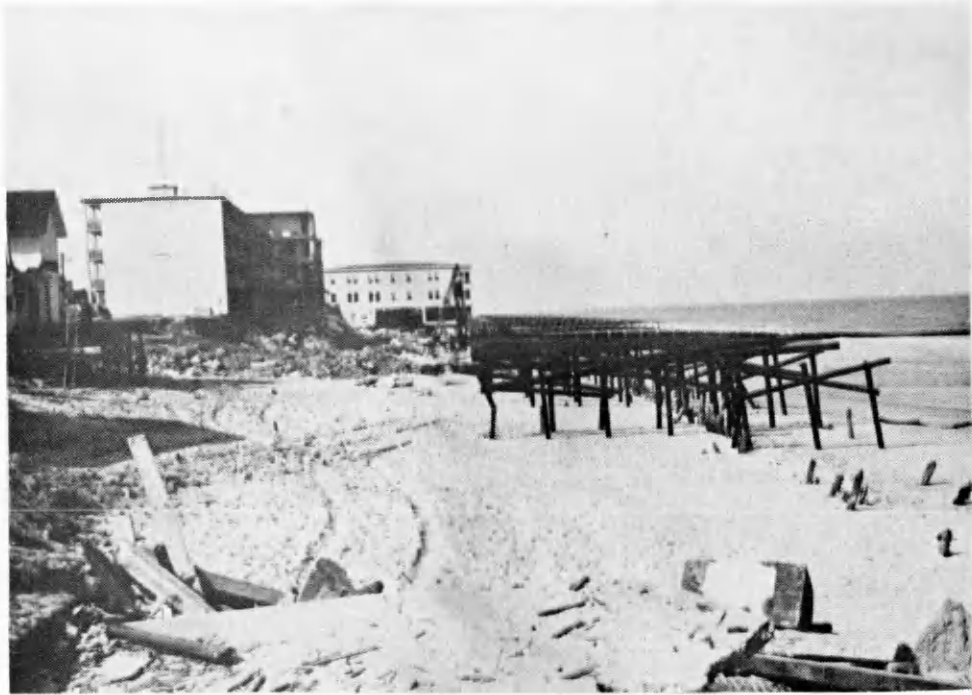
Figure 6. Photograph of property damage at Rehoboth Beach, Del. following the March 1962 storm.
