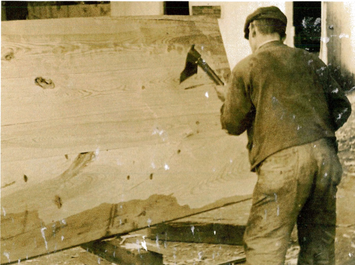
Figure 9. Finishing a log canoe with an adze. Courtesy of the Hampton History Museum, Hampton, Va., 2008.23.7, Detail.
