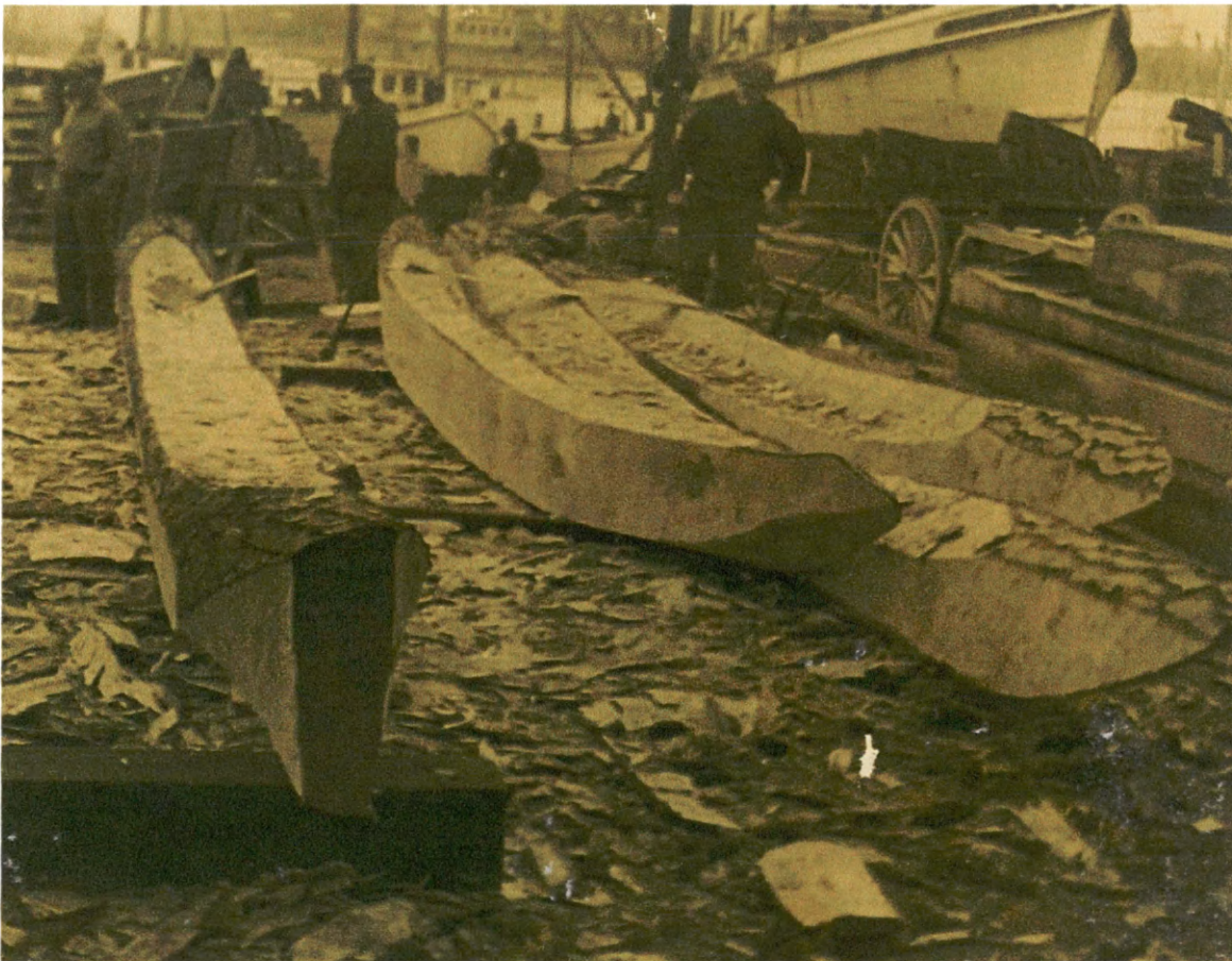
Figure 5. Log canoe construction at Darlings Railway, Hampton. Courtesy of the Hampton History Museum, Hampton, Va., 2008.63.11, Detail.
