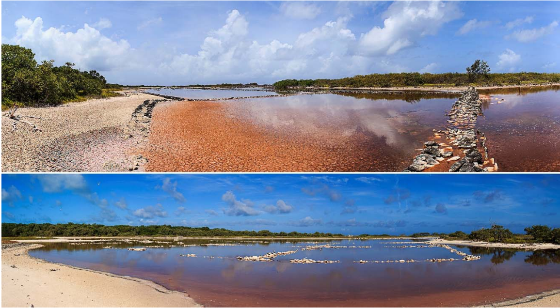
Fig. 5.17. Panorama of the coral stone dikes that crisscross the saltpan of Cayo Sal (photos: José Voglar).
