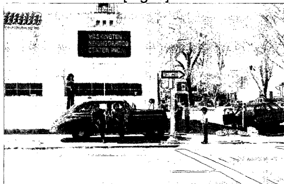
Preparation of Wall For Mural. California State University Sacramento Barrio Art, Organizer. June 1981. Image Courtesy of CEMA at UCSB and Calisphere: http://content.cdlib.org/dynaxml/data/13030/vr/hb5779p1vr/files/hb5779p1vr-FID4.jpg
