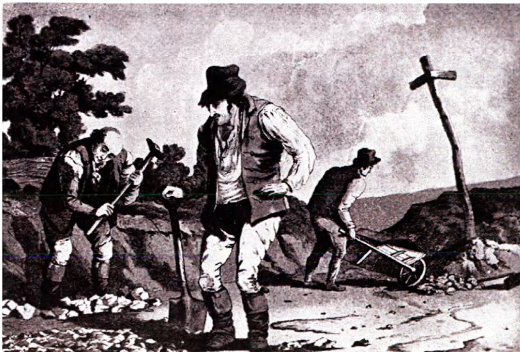
Figure 8. “Stone-Breakers on the Road,” by George Walker, 1800. Early nineteenth-century depiction of a road crew of tithable men in Yorkshire, England, working with a Surveyor of Highways to build and maintain local roads. Road work in Colonial Virginia probably looked similar to this image of highway maintenance in England. (Source: George Walker, The Costume of Yorkshire [London: Longman, Hurst, Rees, Orme and Brown, 1814]. Image reprinted in “The Forgotten ‘Labouring Male Titheable,’” by Nathaniel Mason Pawlett, in Backsights: Essays in Virginia Transportation History, Volume 1: Reprints of Series One, 1972-1985 , by Ann B. Miller, ed. [Charlottesville: Virginia Center for Transportation Innovation & Research, June 2011], 121).
