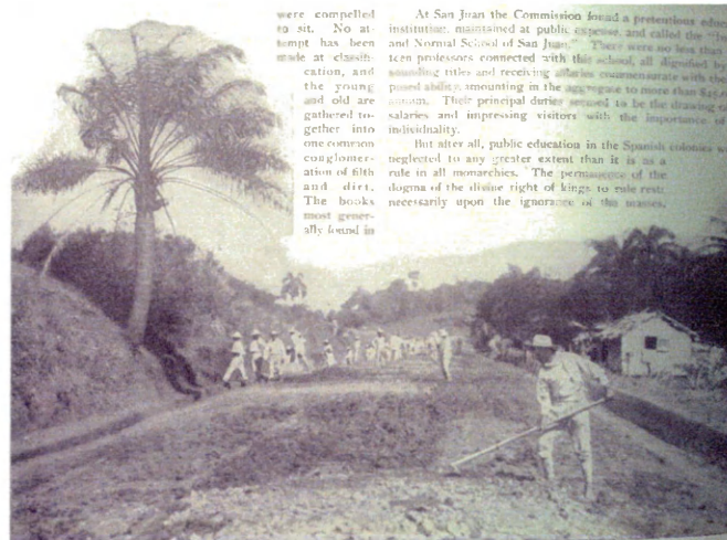
Photo 1. Preparation for macadam paving. (Olivares 1899I:346)
