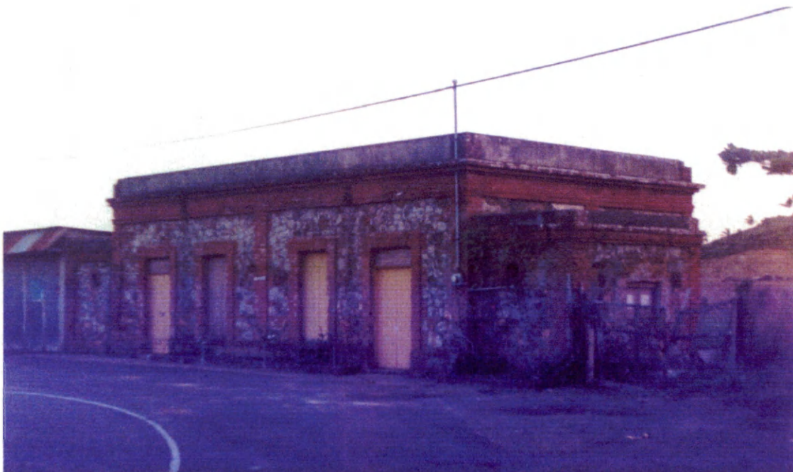
Photo 18. Model #3b casilla, Cayey. Department of Transportation and Public Works.
