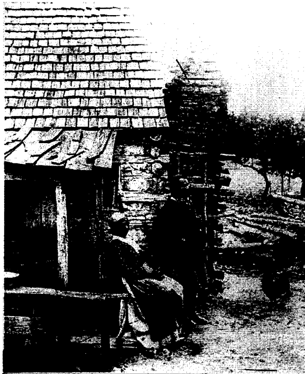
Figure 3.9 – Dwelling of log construction with stick-and-clay chimney, glazed four-panel windows, and covered porch addition, near Richmond, Virginia, 1888. (Valentine Richmond History Center Special Collections and Archives; Virginia Commonwealth University digital collection, negative 1436 http://dig.library.vcu.edu/cdm/singleitem/collection/cook/id/251/rec/225 )
