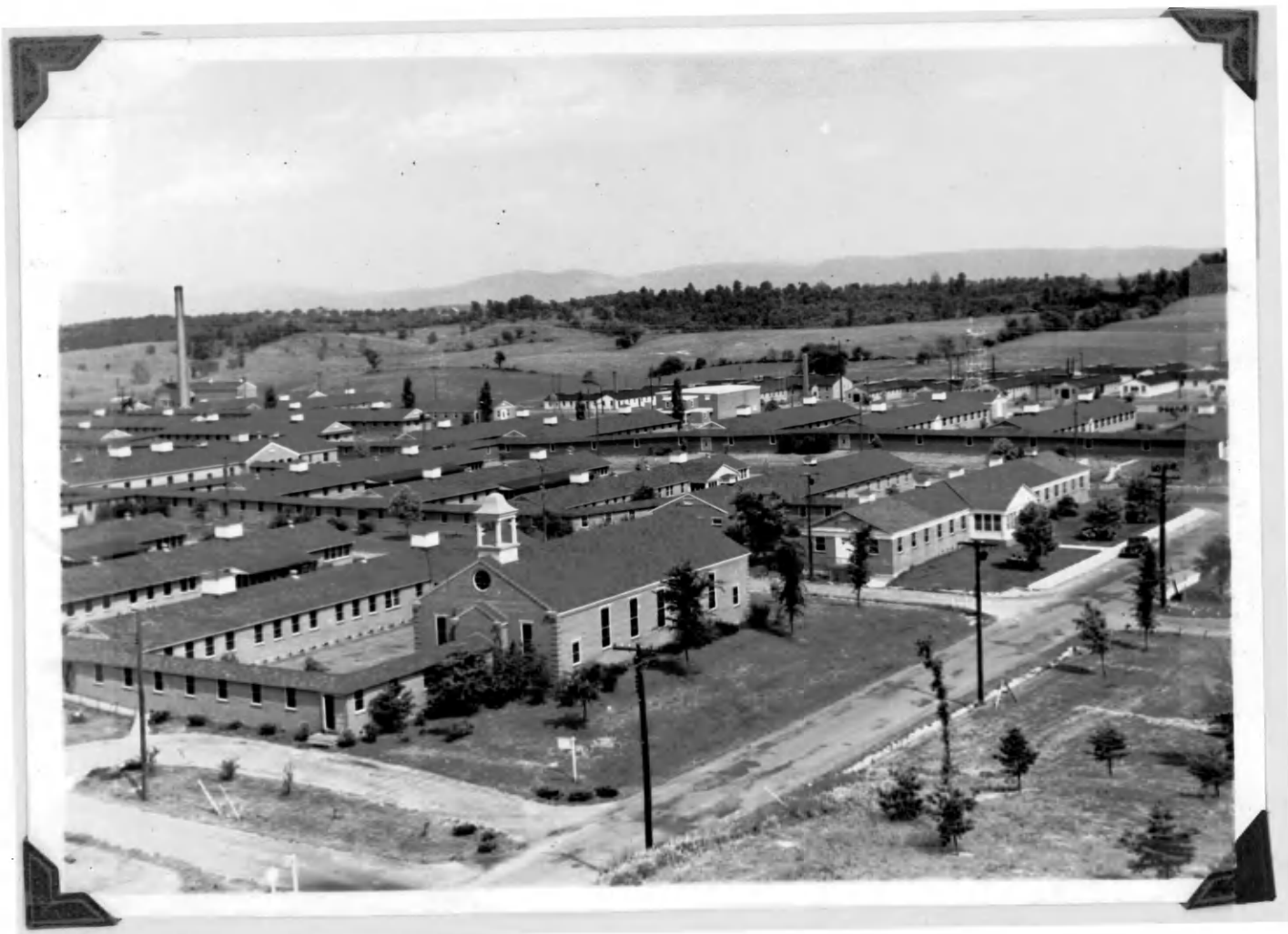
ONE SECTION OF THE PLANT
