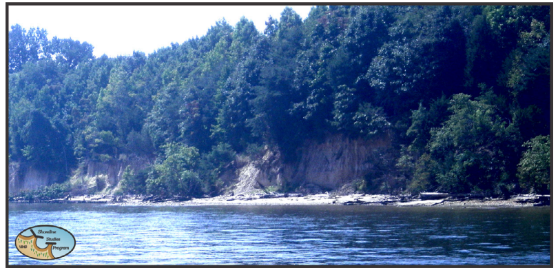
Figure 2-14. Reach 5, eroding banks along the Widewater Peninsula on the Potomac River.
