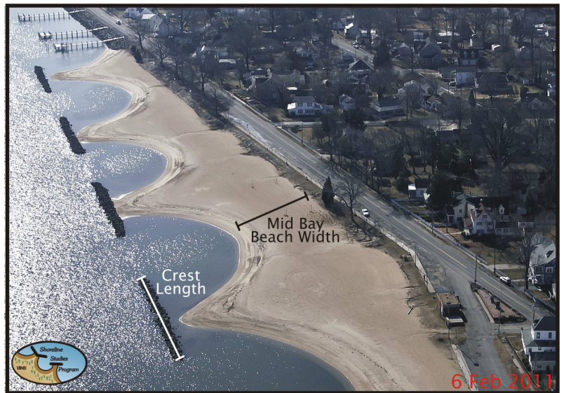
Figure 3-7. Breakwaters at Colonial Beach designed to provide a recreational beach as well as storm erosion protection for the Town.
