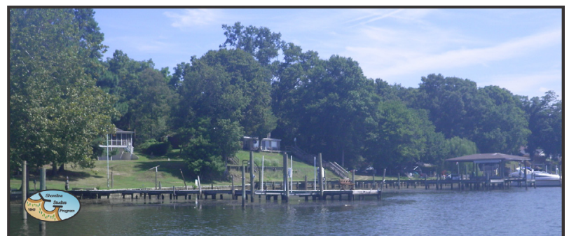
Figure 2-12. Reach 4, shorelines with a low bank and residential landuse. The shoreline has wood bulkheads for protection.
