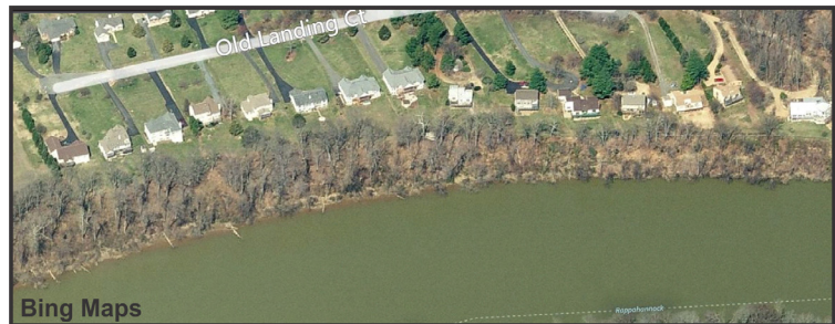
Figure 2-5. Reach 1, Bing map of the eroding high banks along the Rappahannock River in Stafford County.
