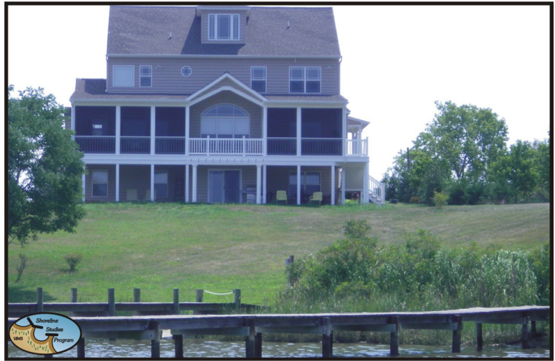
Figure 3-3. Bank grading reduces steepness and will improve growing conditions for vegetation stabilization
