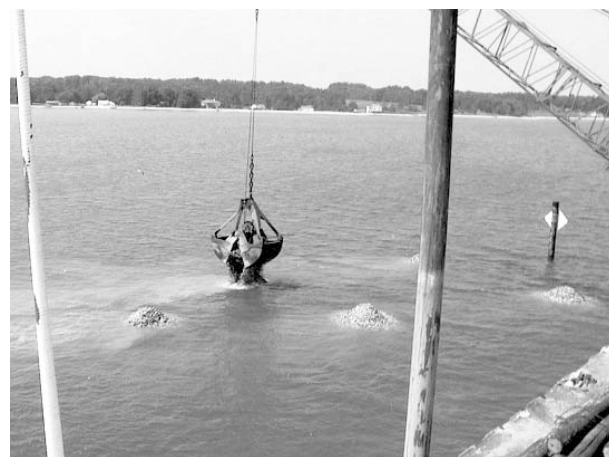
Depositing oyster and clam shells to construct a research reef.
