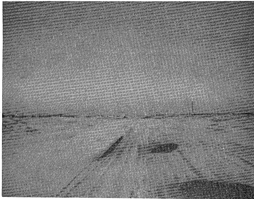
STOP 13b. Privately-owned, paved road of Whalehead Development looking north (top, February, 1976) and ground view of road looking south (bottom, March, 1977). The series of transverse dunes are reasserting their natural geomorphic form under the effects of the westernly winds, resulting in extensive deposition on the road traversing the dunes.
