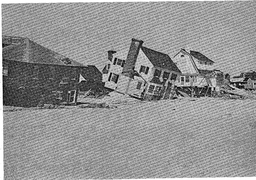
Figure 1. Property damage at Virginia Beach, Va., following the severe March 1962 storm. (Photograph by N. Arthur Pore)
