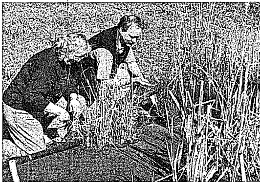
Constructing an artificial marsh
