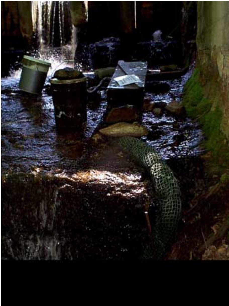
Figure 3. The Irish ramp at Clark's Millpond (Coan River). The green tube in the foreground was initially used as the modified ramp extension. In 2004, the "tube" was replaced with \frac{1}{4} " Delta knotless nylon placed in layers in the same location.
