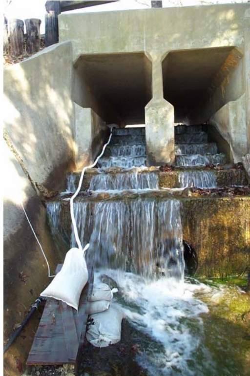
Figure 6. Example of an Irish eel ramp used in this study. The arrows indicate the flow of water as well as eel movement.
