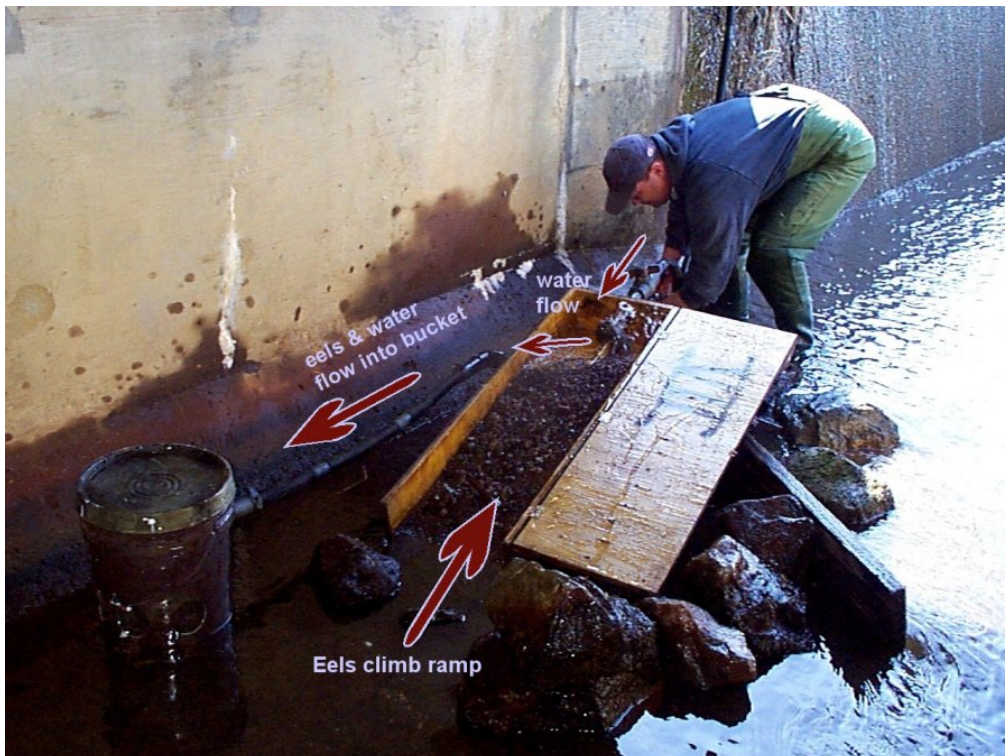
Figure 6. Example of an Irish eel ramp used in this study. The arrows indicate the flow of water as well as eel movement.
