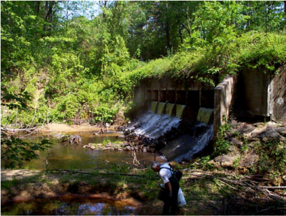
Figure 4. View of Kamp's Millpond spillway and tailrace.
