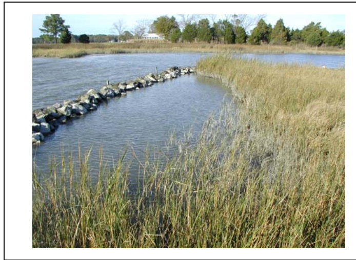
Figure 7. Erosion of the marsh edge continued at one section of this project where the offset distance of the marsh sill was greater than 10 feet. There was no erosion observed where the same sill was closer to the marsh edge.
