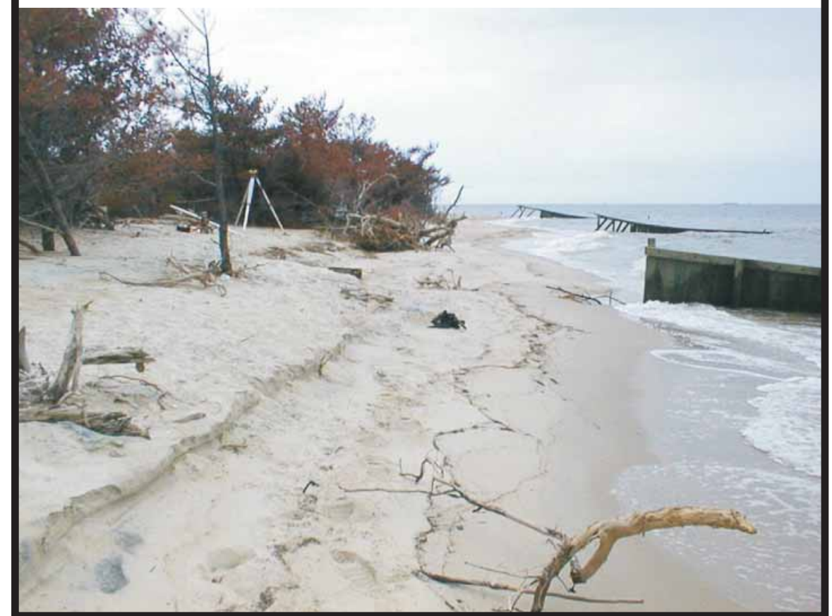
Figure 14-3. Impact of Hurricane Isabel on NI42's structures.
