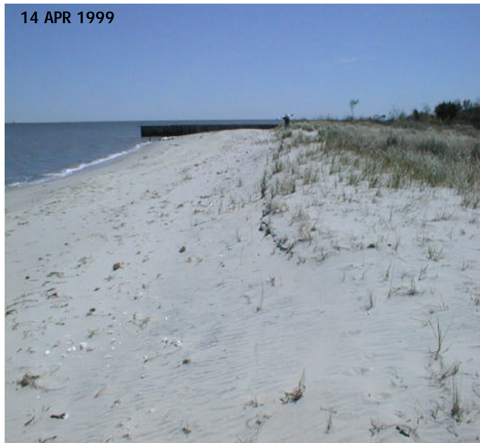
Looking south at Garden Creek jetties.
