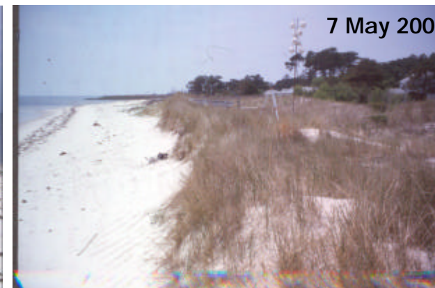
Looking south along the primary dune crest at MA 3.
