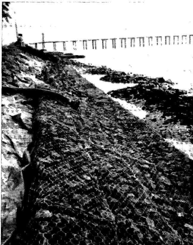
Figure 22 – Gabion revetment.
