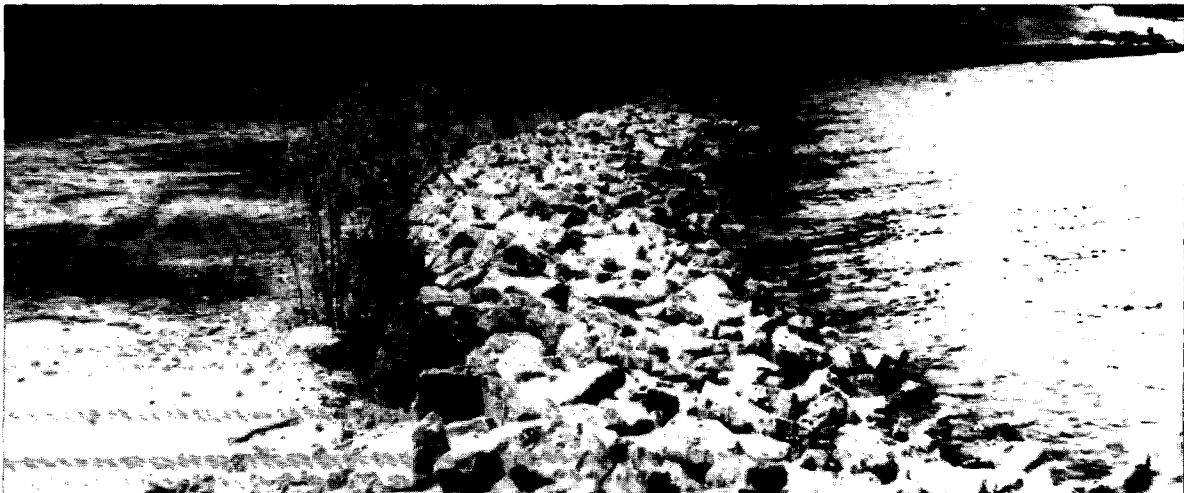
Figure 15 — Concrete seawall (top). Figure 16B (bottom) small riprap revetment. Figure 16A (middle) riprap revetment.
