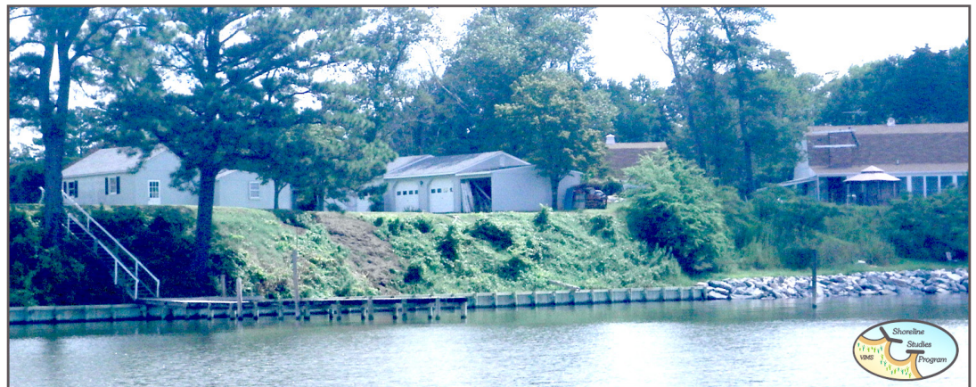
Figure 2-10. Eroding upland banks with residential properties on Gloucester's York River that have been hardened with bulkheads and revetments.
