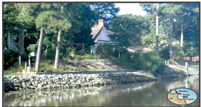
Figure 2-13. Shoreline hardening in the low fetch environment of Sarah Creek.
