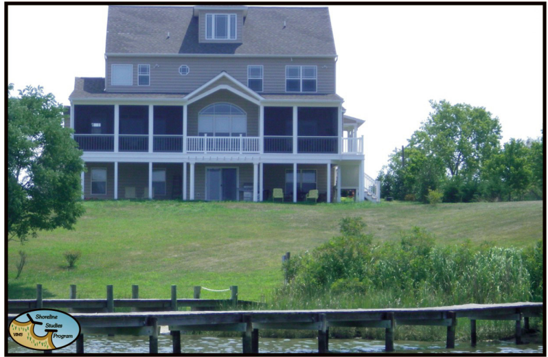
Figure 3-3. Bank grading reduces steepness and will improve growing conditions for vegetation stabilization.
