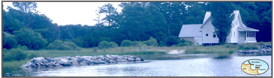
Figure 2-9. Breakwaters at Fox Creek in Gloucester County.
