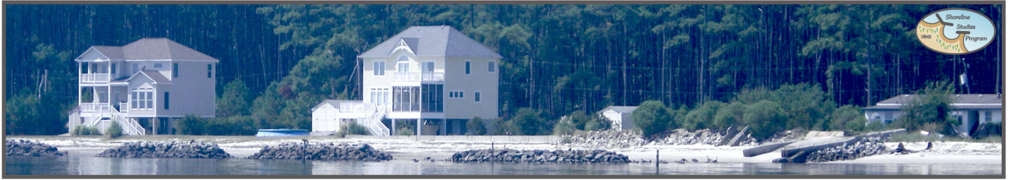
Figure 2-19. North River residential properties with a low bank and breakwaters for shore protection.
