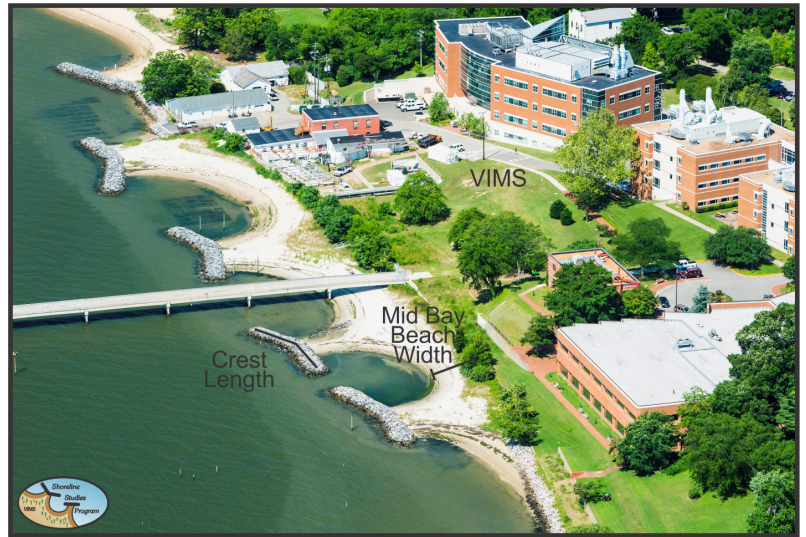
Figure 3-7. Breakwaters at VIMS designed to provide a wide beach for storm erosion protection at the campus.
