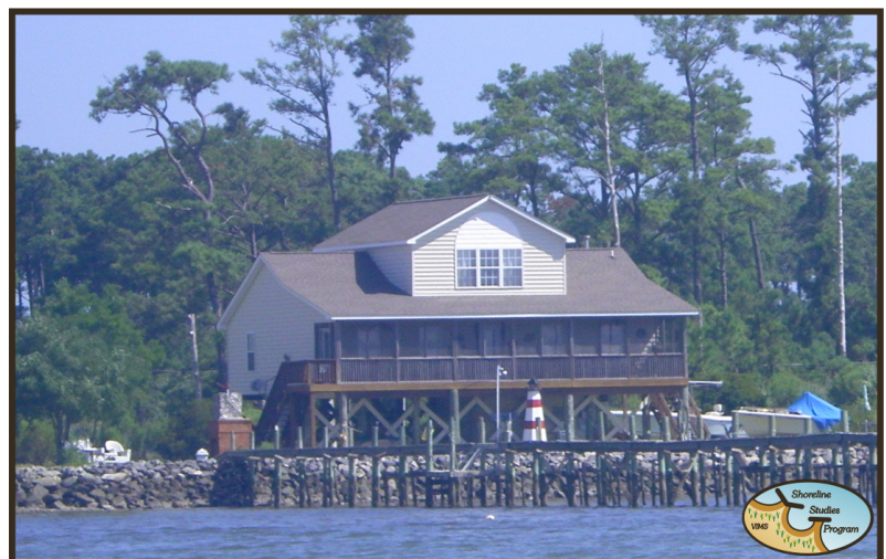
Figure 2-15. Raised houses and shore protection along shorelines that have been significantly impacted by storms.
