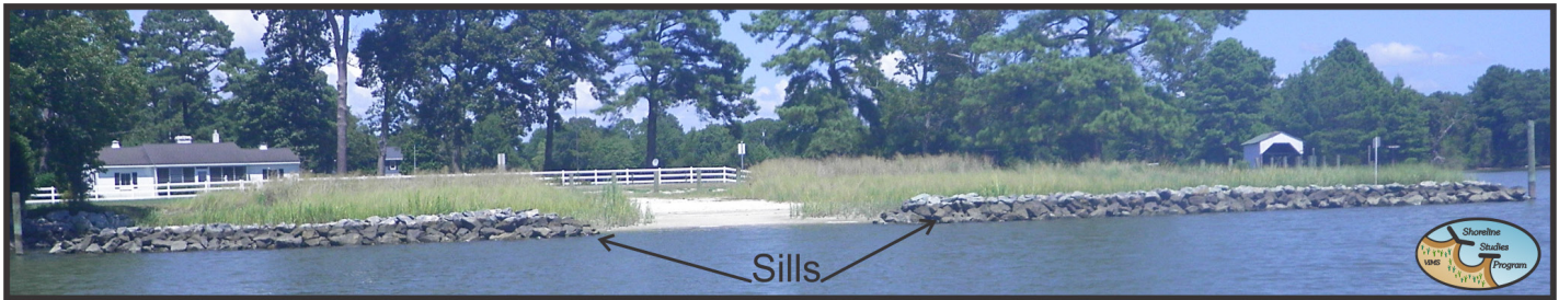
Figure 2-17. Living Shoreline sills at Jones Wharf on Free School Creek.
