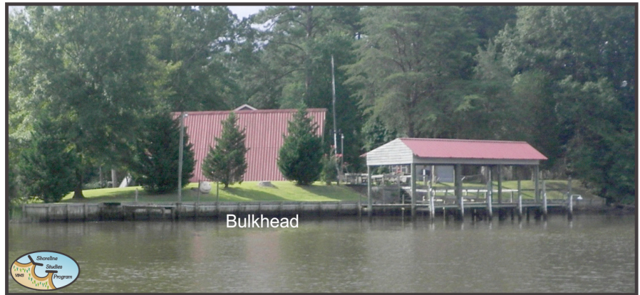
Figure 2-6. Low bank and bulkheading on the Poropotank River.
