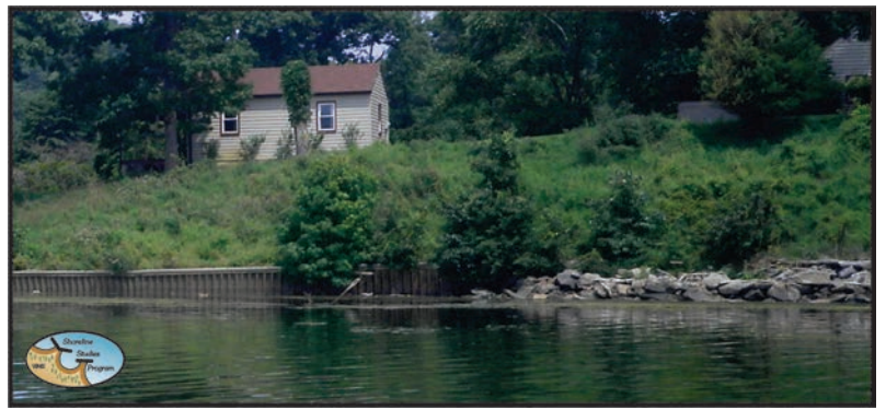
Figure 2-6. Shore protection along eroding banks of Belmont Bay.
