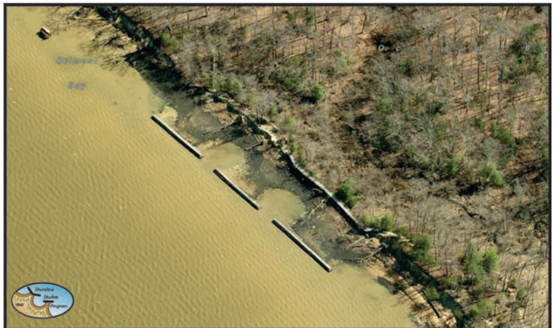
Figure 2-8. Gabion structures that are acting as breakwaters along Mason Neck State Park. From Bing Maps.
