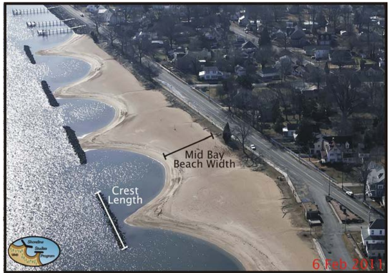
Figure 3-8. The breakwaters at Colonial Beach provide a wide recreational beach as well as storm erosion protection for the residential upland. These structures were installed in 1982.
