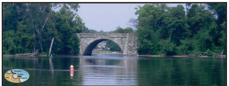
Figure 2-16. The fixed entrance to Little Hunting Creek.
