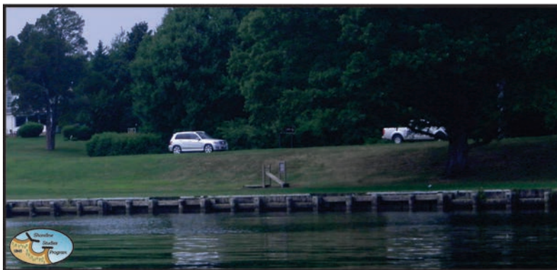
Figure 2-17. The George Washington Memorial Parkway runs along the shoreline in Reach 3.
