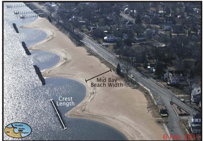
Figure 3-8. The breakwaters at Colonial Beach, Virginia provide a wide recreational beach as well as storm erosion protection for the residential upland. These structures were installed in 1982.
