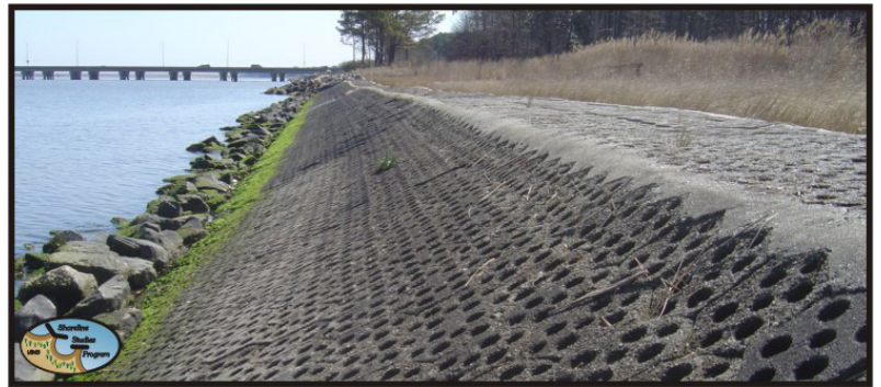
Figure 2-6. Experimental Seabee revetment. Photo date, 22 Mar 2009.
