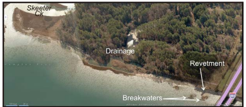
Figure 5-6. Tidewater Community College shoreline east of Interstate 664.
