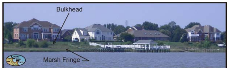
Figure 2-8. Houses along a high bank on the Nansemond River are protected by a marsh fringe and bulkheads constructed at the boundary between the upland and marsh.
