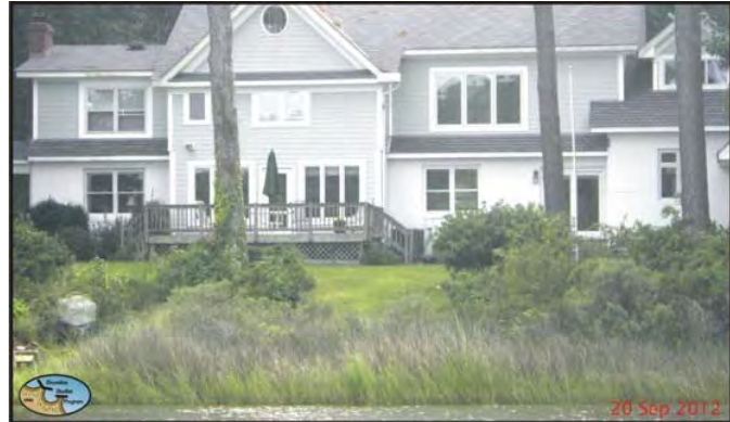
Figure 3-2. Maintaining and enhancing the riparian and marsh buffers can maintain a stable coastal slope.
