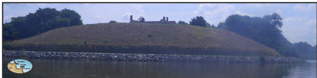
Figure 2-7. Armored shoreline at City Point at the confluence of the Appomattox and James Rivers.
