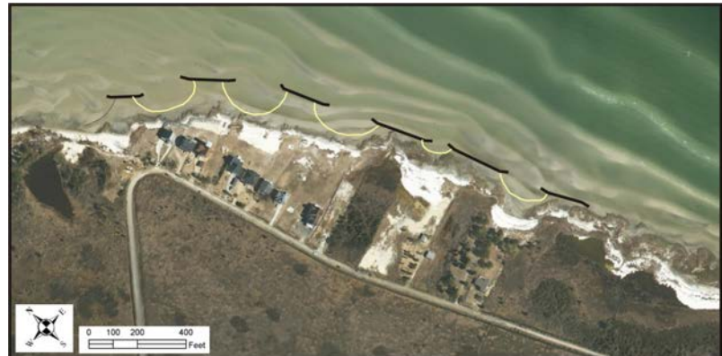
Figure 5-7. Site-specific application of the Shoreline Management Model recommendation for Bay Tree Beach. The breakwater system will stabilize the shoreline, provide shore protection, and create a recreational beach. The sills will stabilize the marsh.
