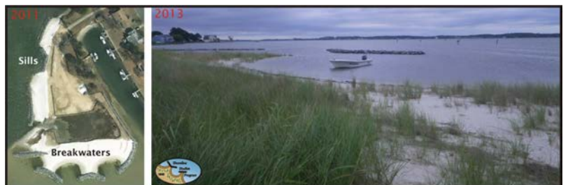
Figure 3-10. Headland breakwaters at the confluence of Cabin Creek and the Poquoson River. These structures were built relatively closely-space to provide a recreational beach as well as to protect the upland. Left: A 2011 Virginia Base Mapping Program image shortly after installation. Right: Photo taken in July 2013. Planted beach grasses have thrived at the site.
