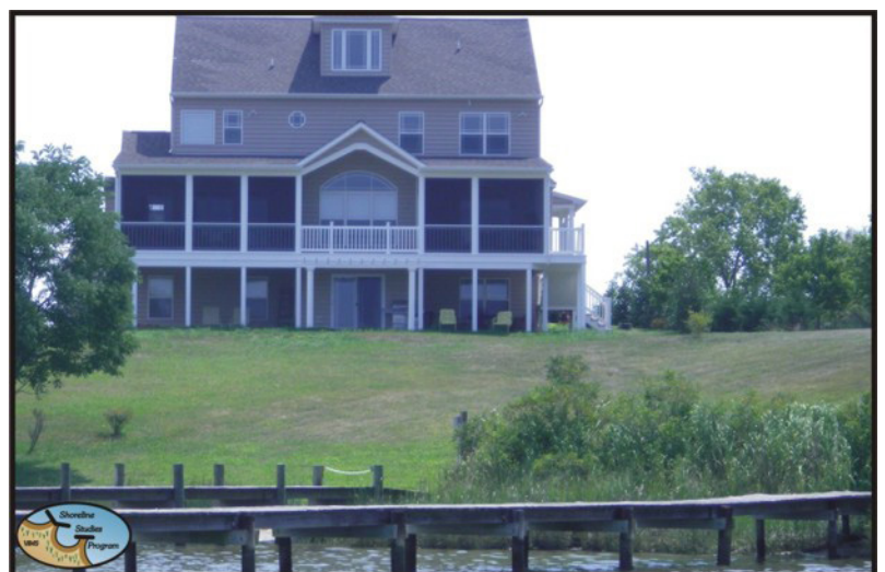
Figure 3-3. Bank grading in Westmoreland County reduces steepness and will improve growing conditions for vegetation stabilization.
