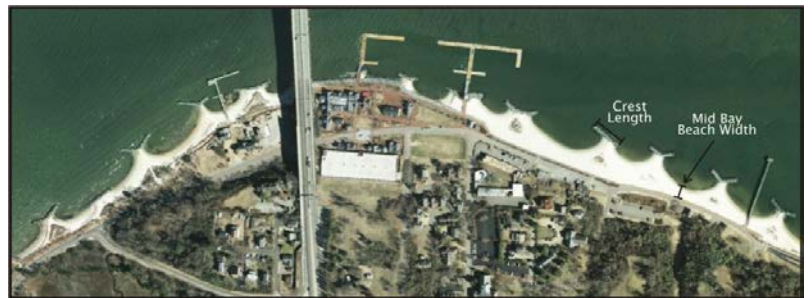
Figure 3-9. The breakwaters at Yorktown provide a wide recreational beach as well as storm erosion protection for the business district. These structures were phased in beginning in 1994. 2011 Virginia Base Mapping Program Image.
