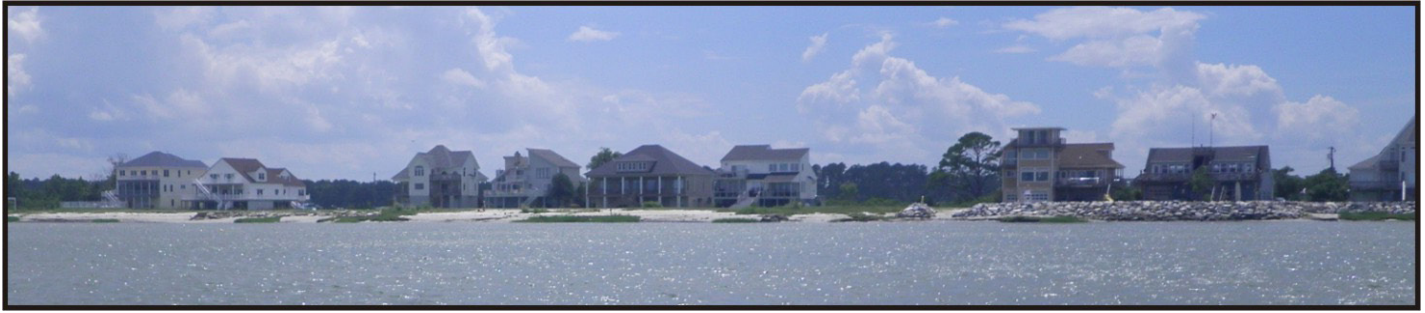
Figure 5-5. The Bay Tree Beach shoreline consists of eroding marsh headlands and sand washover. A revetment was constructed along the shoreline.
