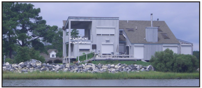
Figure 2-8. Low upland bank in a residential area that has a rock revetment for shore protection behind a fringe marsh
