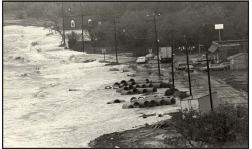
Figure 3-8. Photo taken at Yorktown during a spring storm. The low coast was easily overwashed.
