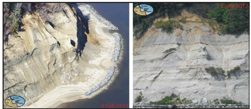
Figure 3-7. High sills built along Westmoreland State Park's high energy, high bank shoreline. The material that slumps from the bank will be caught behind the sills and stabilize the base of the bank by protecting it from wave attack. A more recent photo shows that the slump material is starting to become vegetated.
