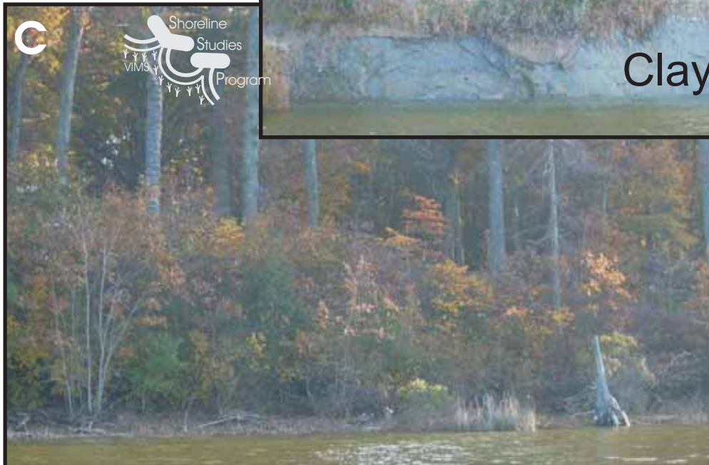
Figure 5-2. Site 349, as identified in the Mathews County Shoreline Management Plan, on the Piankatank River. A) The eastern end of the site is low, wooded and eroding. B) the high banks along the site are vertically-exposed and eroding. C) The western end of the site also is low, wooded and eroding.
