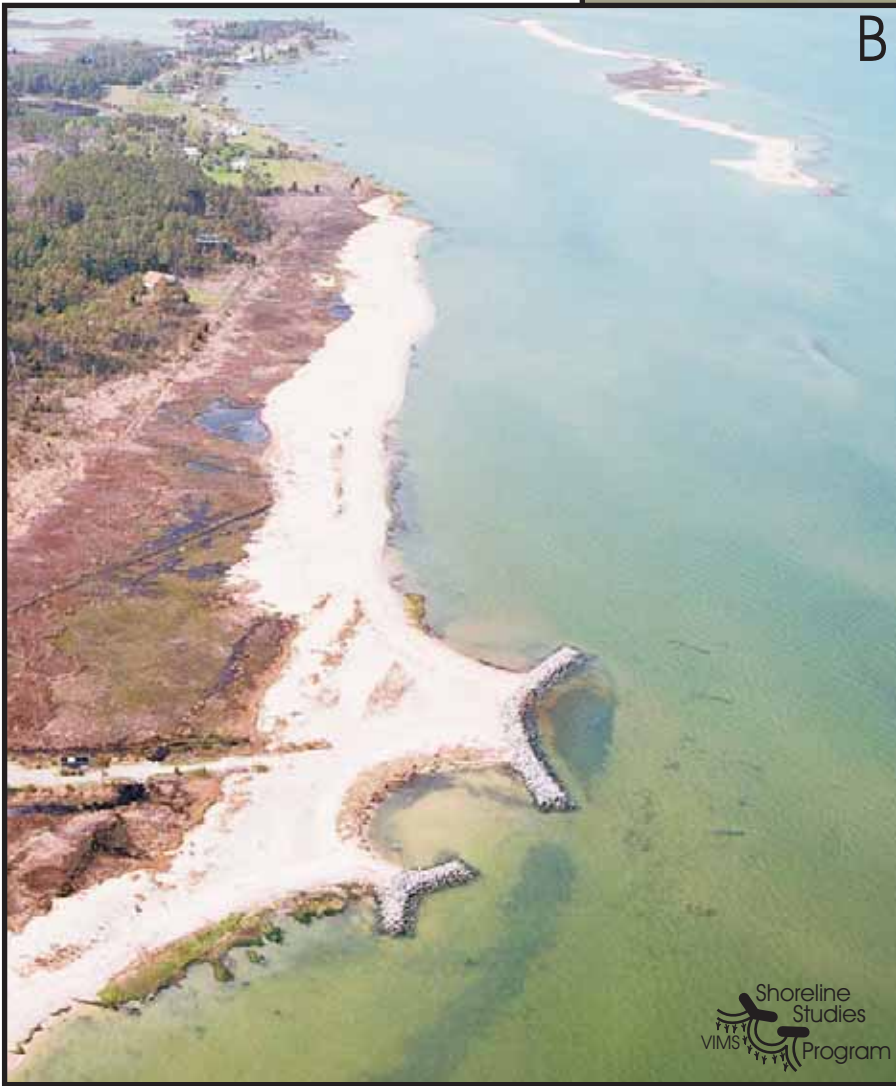
Figure 3-5. Aerial photos of A) Drummond Field breakwaters (June 30, 2005) on the James River, and B) Festival Beach on Chesapeake Bay (April 21, 2010). While the physical characteristics of each site differ, the goals are the same: protect the upland bank/marsh with a wide recreational beach.
