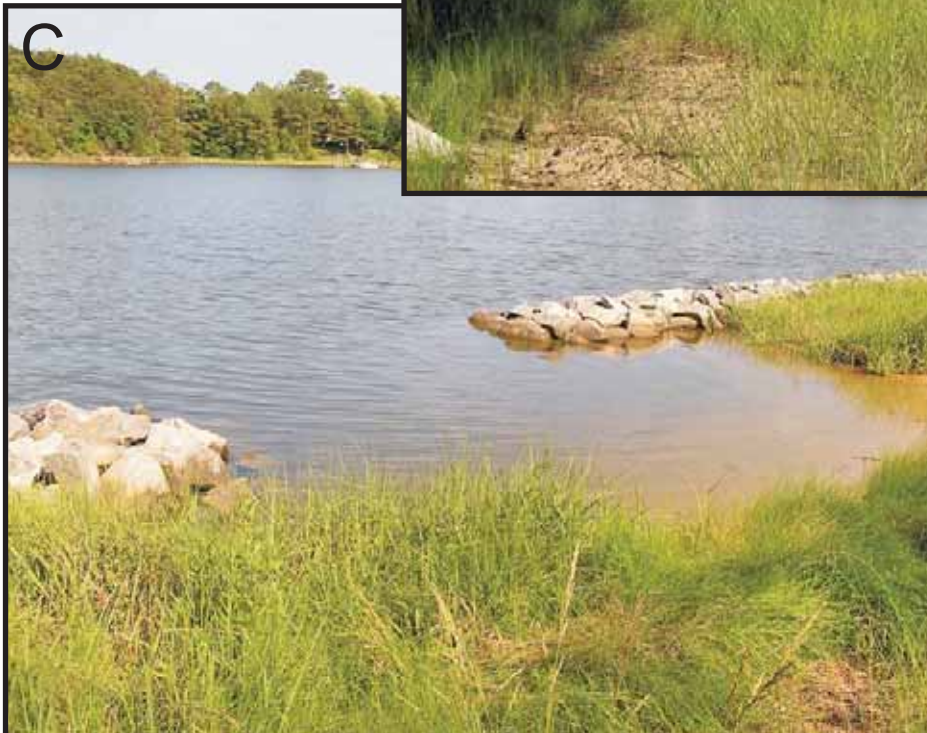
Figure 4-3. Foxx site photos. A) Before construction, the upland bank was undercut and only a small intermittent marsh fringe existed. B) After construction, a wide, marsh fringe and graded bank stabilized the site. C) Gaps in the sill allow waves in, reducing the width of the marsh there.
