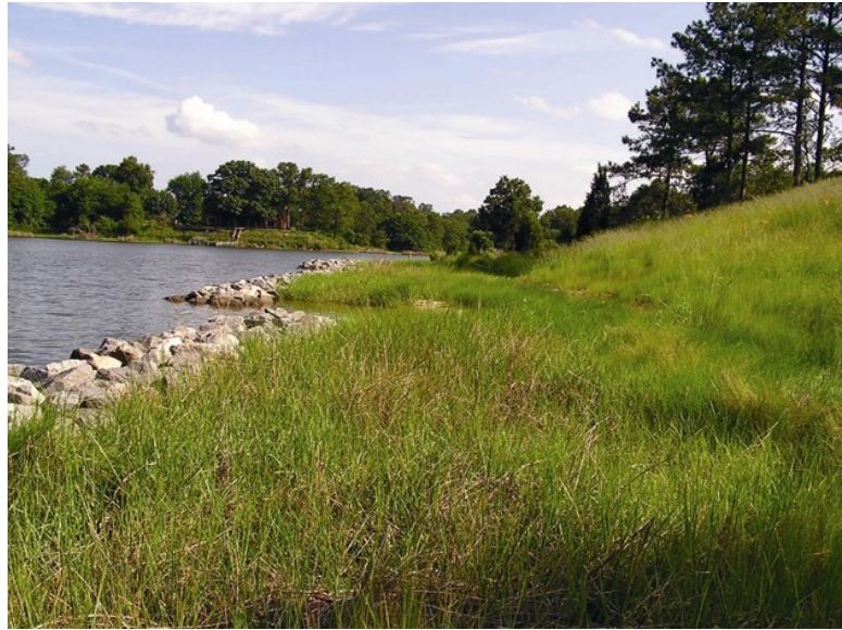
Figure 9.1. Example of a living shoreline installed as an alternative to an exclusive revetment erosion control structure. Photo credit: Karen Duhring.
