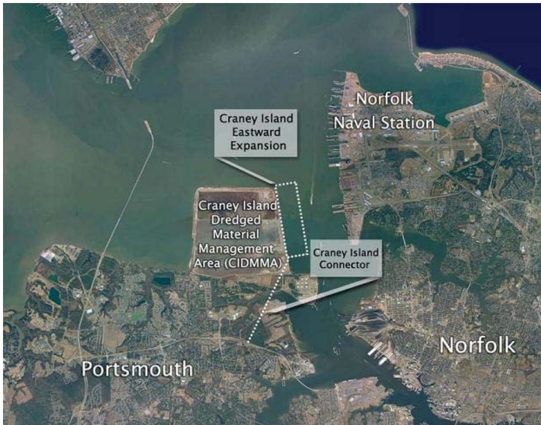
Figure II.1. Aerial view of CIDMMA, located along James River south bank in Portsmouth, VA
