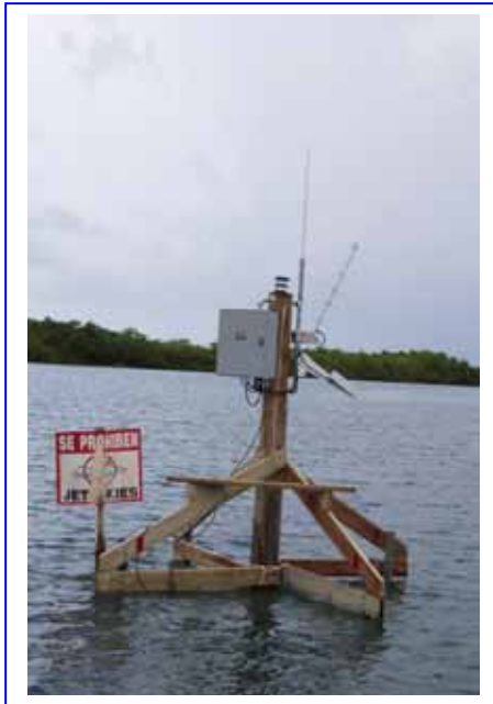
Figure 5.40 One-column structure (Source: Jobos Bay, NERR)
