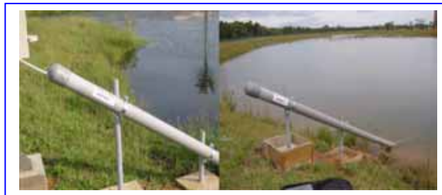
Figure 5.52 Cement foundation, pipe, pipe fasteners mounting system (Source: Universiti Sains Malaysia)
