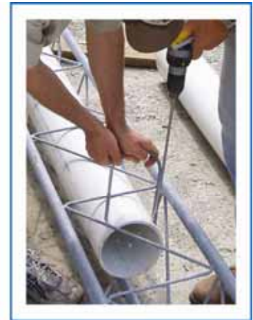
Figure 5.29 Drilling holes to place U-bolts.
