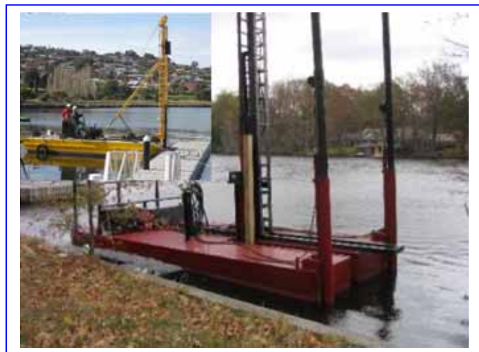
Figure 5.5 Small pile driving work barge (Source: ASD Pty Ltd., Marine Pile Drivers)
