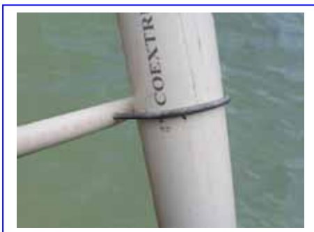
Figure 5.15 The Transverse PVC is fastened to the structure leg by a U-Bolt
