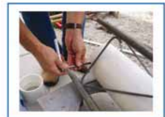
Figure 5.27 Threading top holes.
