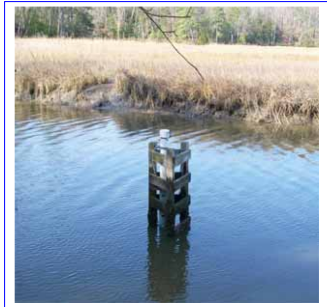
Figure 5.41 Three-column structure (Source: Taskinas Creek, NERRVA)
