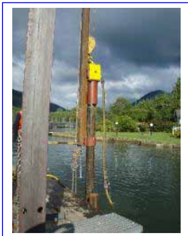
Figure 5.4 Drop hammer (Source: Whatcom Waterfront Construction)
