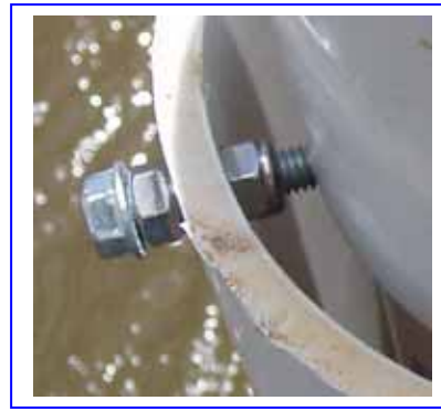
Figure 5.18 Close-Up view of a bolt-double nut
