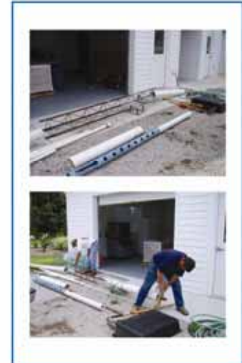
Figure 5.26 Inserting 6 foot long 6 in PVC pipe into the antenna tower.
