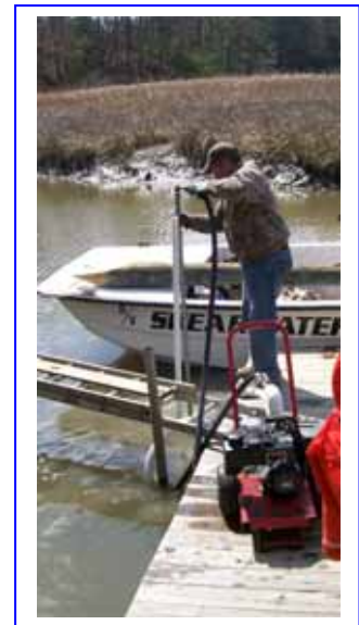
Figure 5.8 Jetting initial hole
