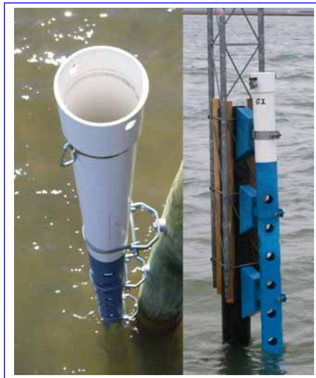
Figure 5.12 View of different methods used to attach the guard-pipe to the pile.
