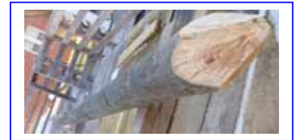
Figure 5.6 View of pile bottom
