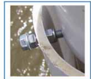
Figure 5.28 Hex head bolts with two lock nuts.
