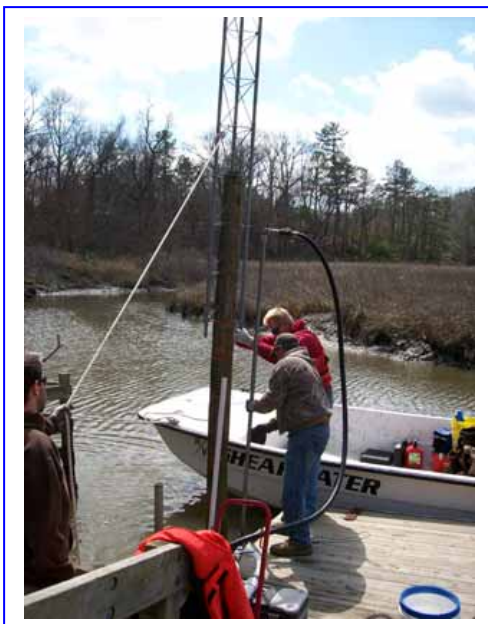
Figure 5.9 Jetting process
